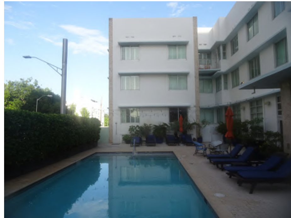
INTERIOR COURTYARD LOOKING WEST- 01.14.2022
