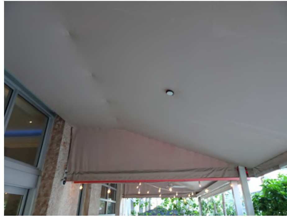
FRONT PORCH FABRIC AWNING- 01.14.2022
