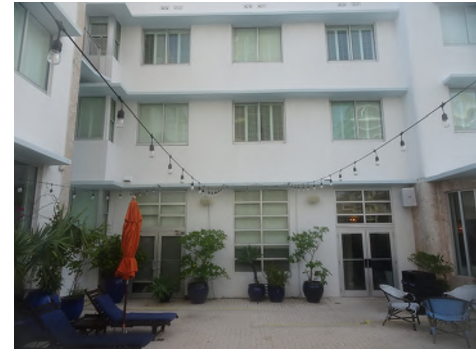
INTERIOR COURTYARD LOOKING NORTH 01.14.2022
