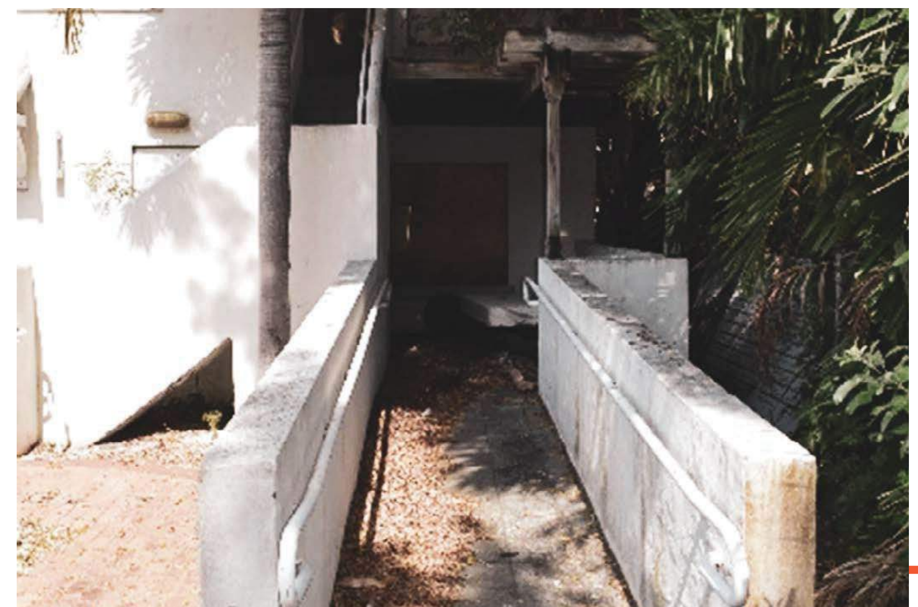
Front Yard Detail ACCESSIBLE RAMP (NON-ORIGINAL, TO BE REMOVED)
