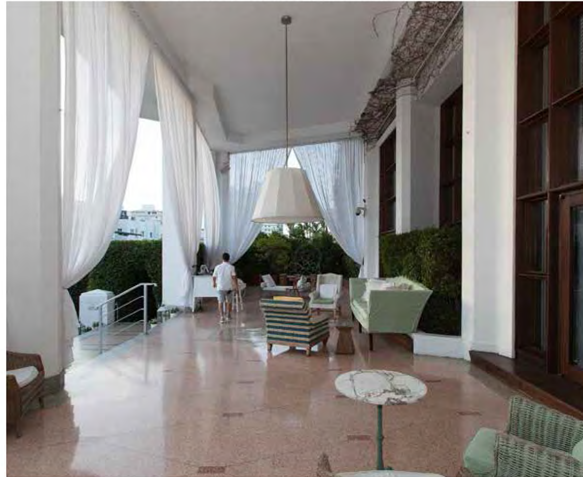
EXISTING TERRAZZO FLOORING
