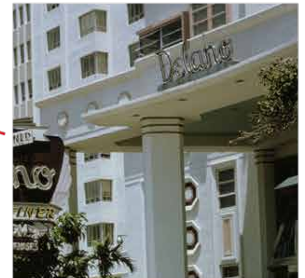
Original signage location to be replicated
