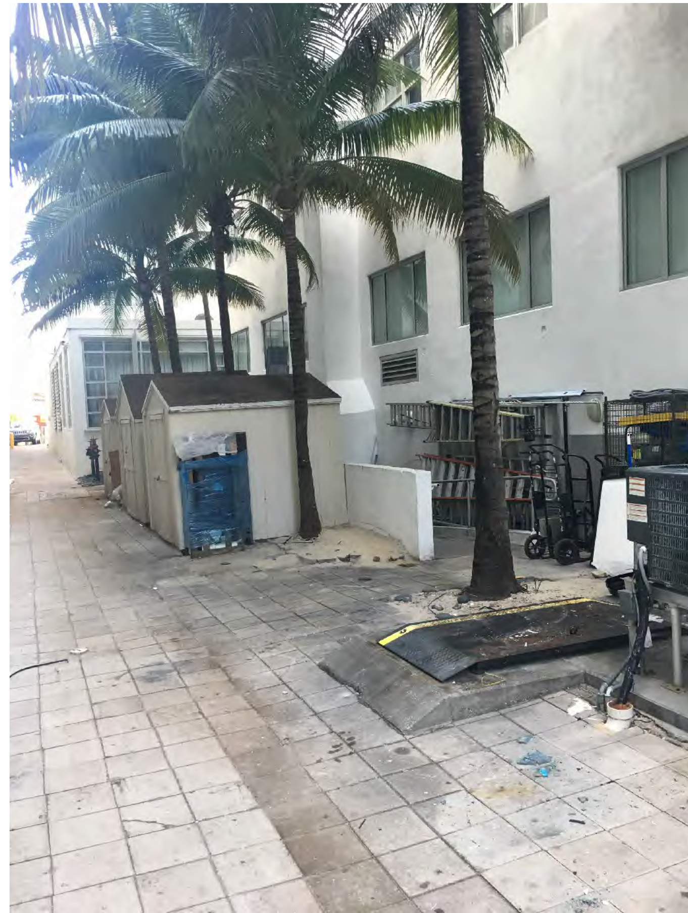
GENERAL VIEW SHOWING EXTERIOR BUILDING SOUTH ELEVATION
