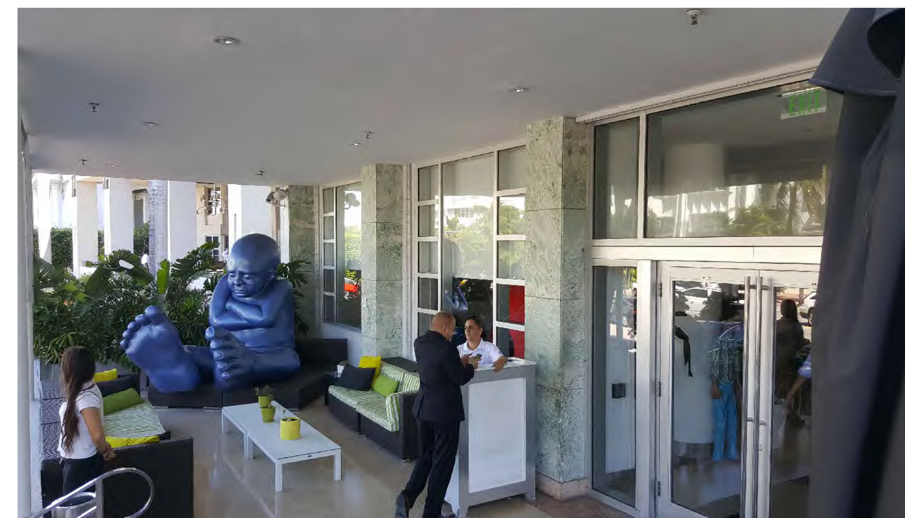
5 VIEW OF EXISTING MAIN ENTRY DOOR AREA
