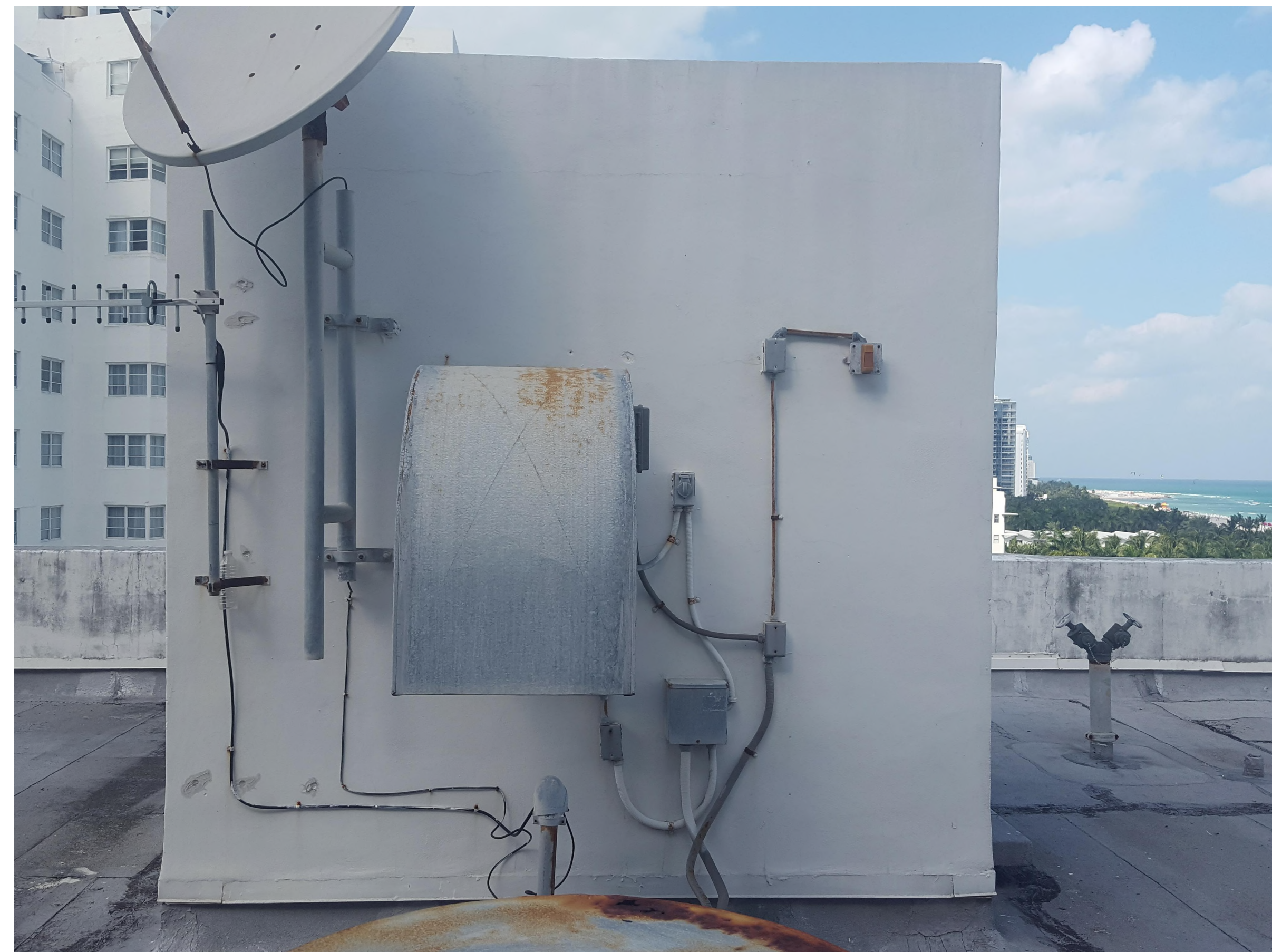
VIEW OF THE EAST ELEVATOR ROOF OVER-RUN
