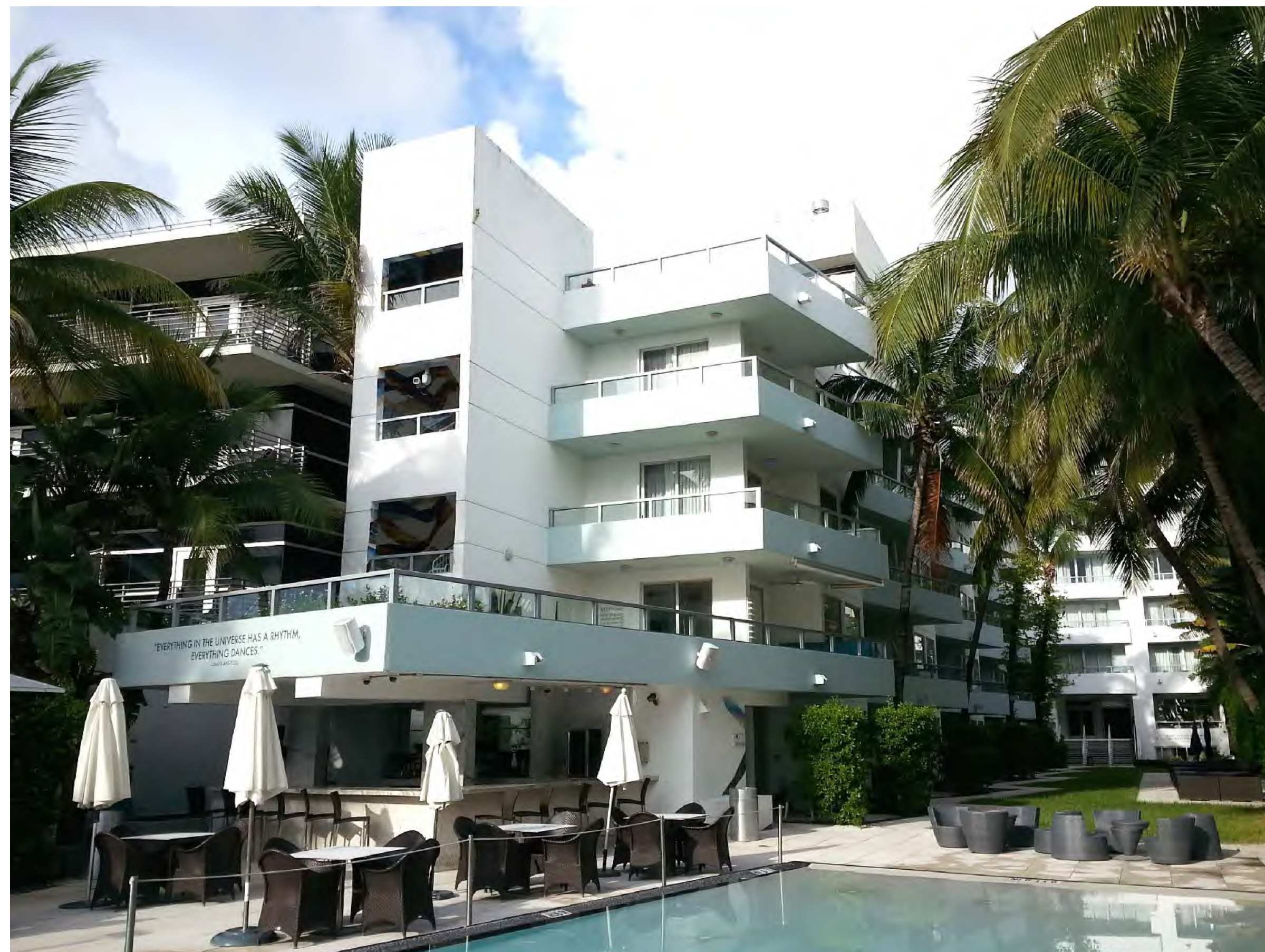
VIEW OF BUNGLOWS AND INTERIOR COURTYARD FROM POOL DECK
