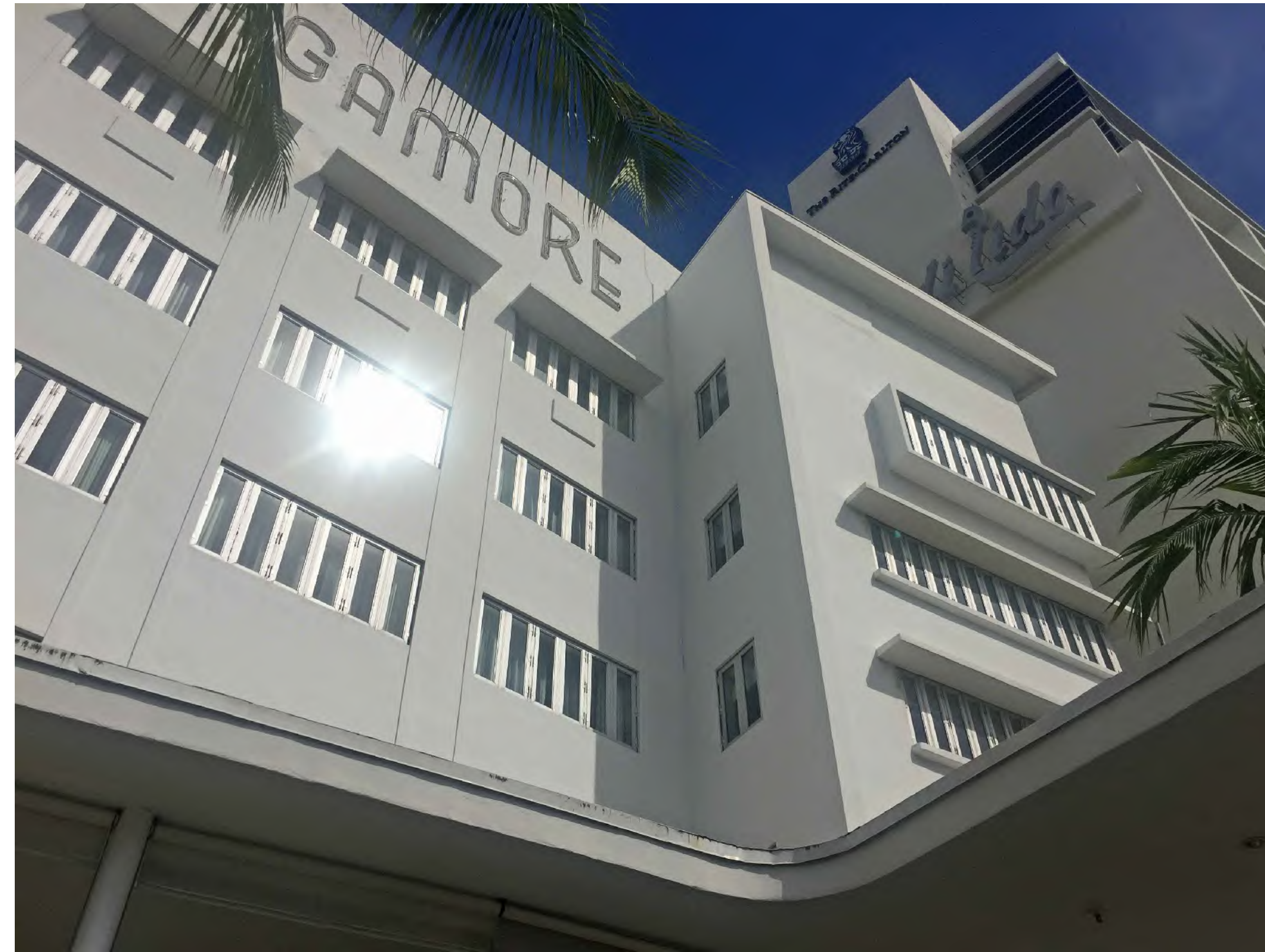
DETAIL OF MAIN BUILDING FRONT FACADE FROM COLLINS AVENUE
