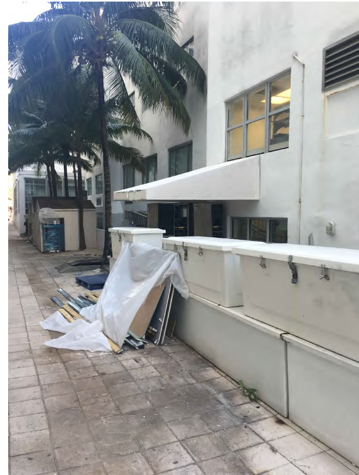
GENERAL VIEW SHOWING EXTERIOR BUILDING SOUTH ELEVATION
