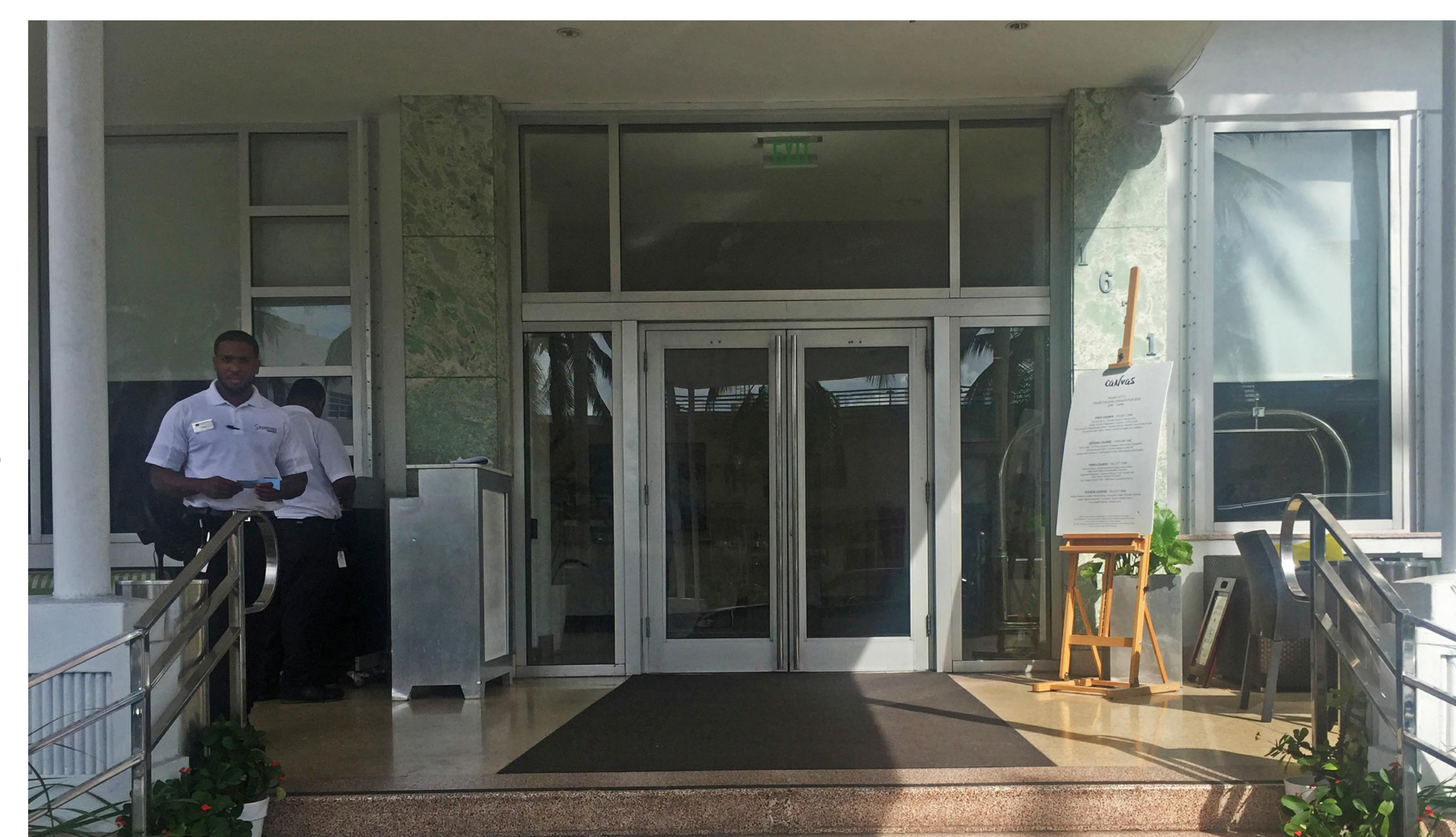
7 VIEW OF EXISTING MAIN ENTRY DOOR
