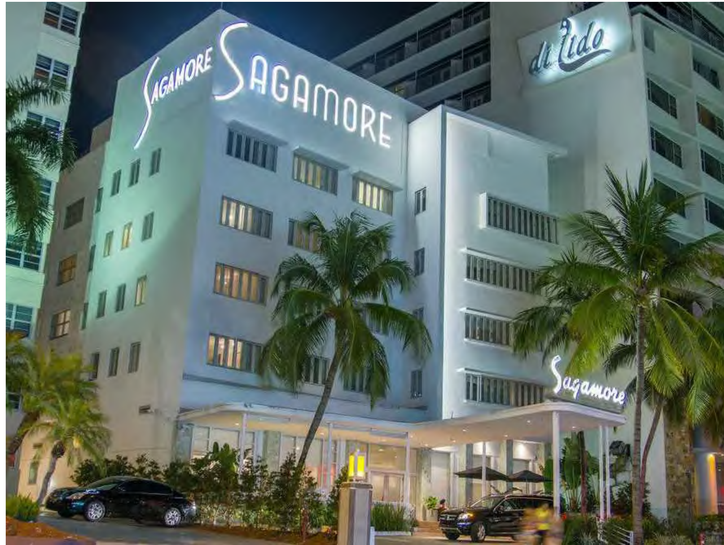
VIEW OF MAIN BUILDING FRONT FACADE FROM COLLINS AVENUE
