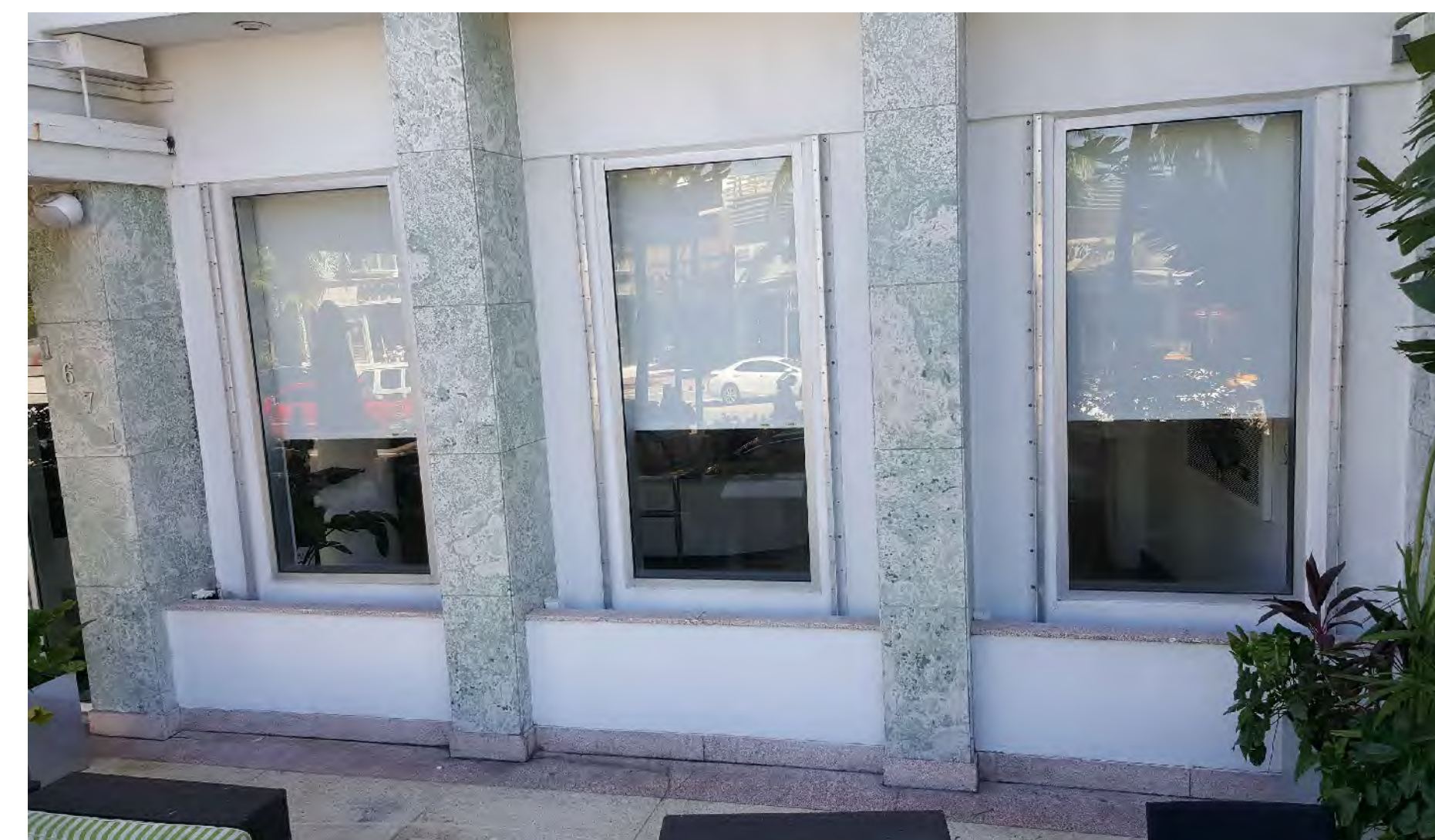
6 VIEW OF EXISTING FIXED GLASS WINDOW
