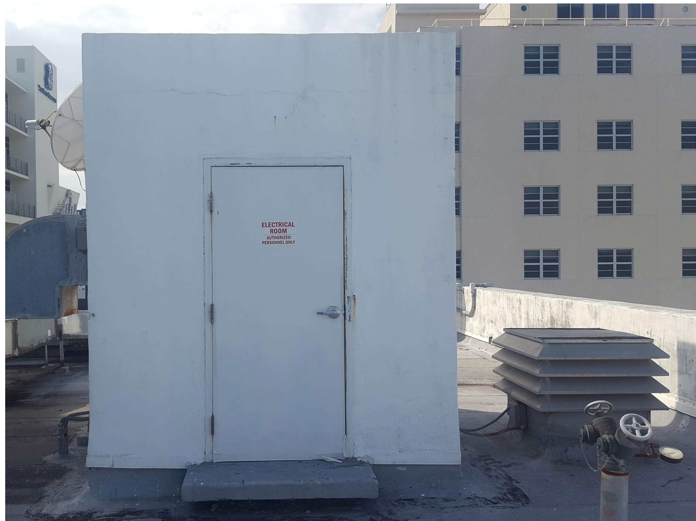
VIEW OF THE EAST ELEVATOR ROOF OVER-RUN
