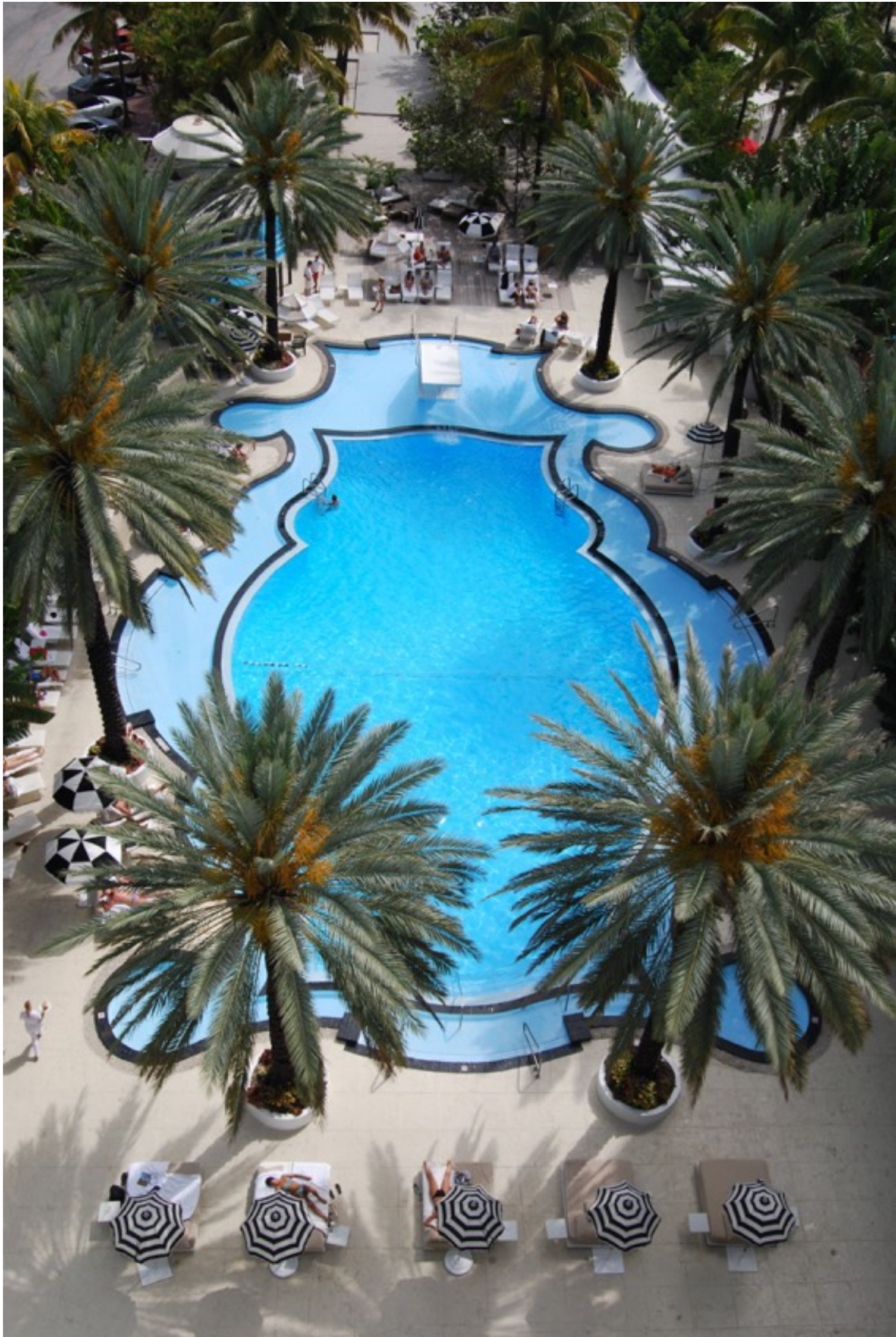
C - 2013 PHOTO ABOVE SHOWS INNER DEEP POOL AND OUTER WADING POOL (FORMER WALKWAY) (14) WITH ALL FORMERLY RED BRICK COPING PAINTED BLACK.
