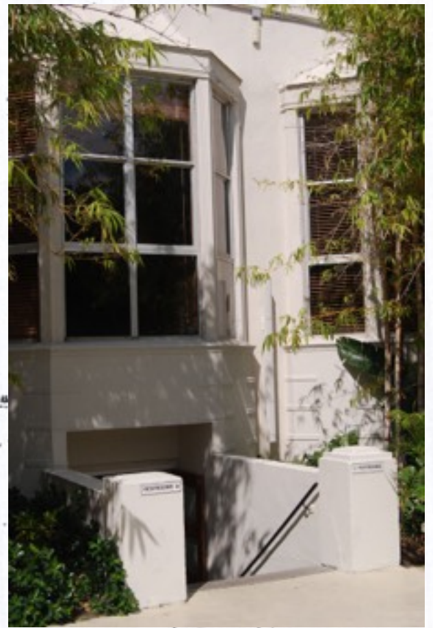
POOL RESTROOM ACCESS BENEATH DINING ROOM (14)
