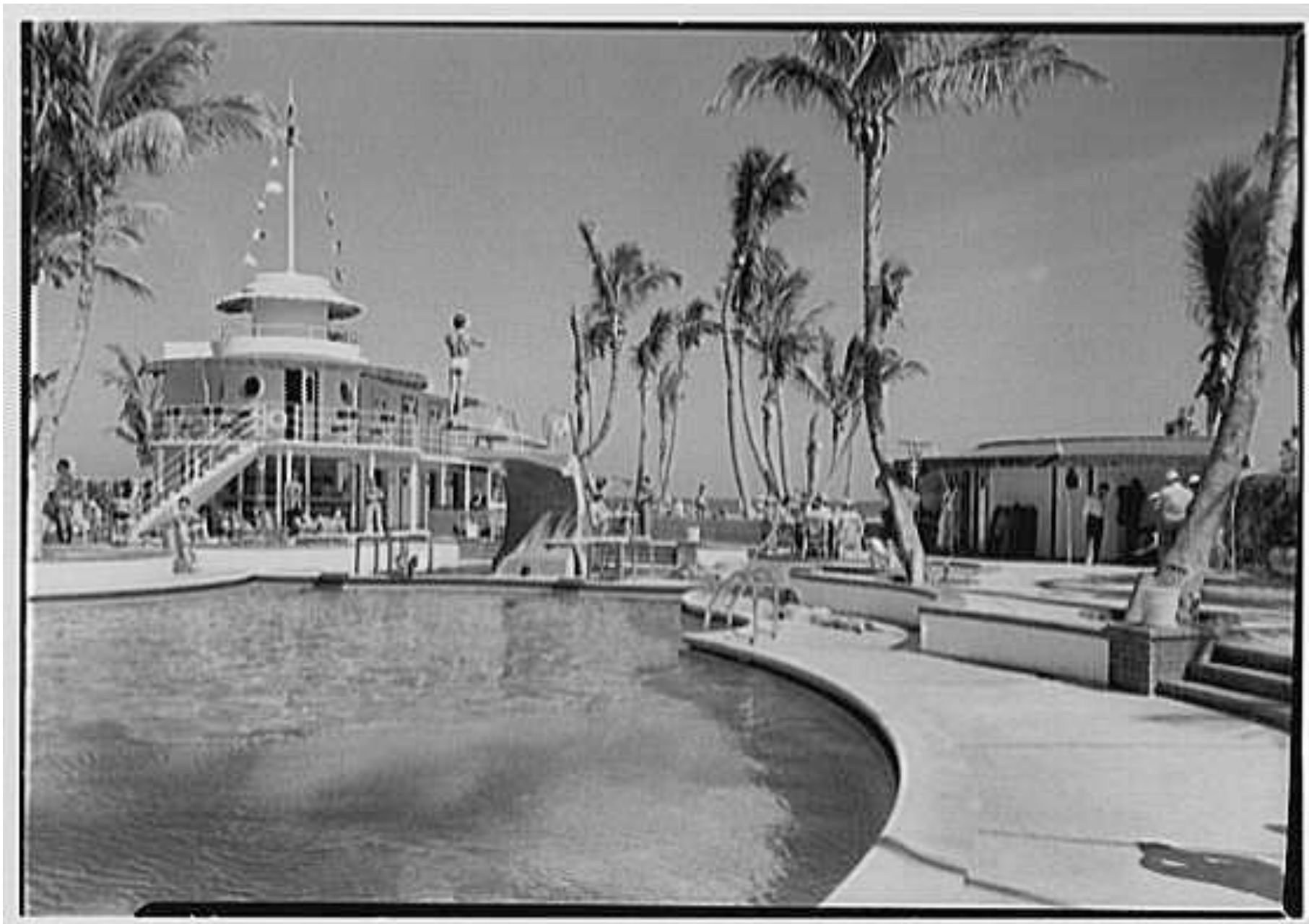
A - ORIGINAL DEEP POOL WITH CONCRETE COPING AROUND POOL AND RED BRICK COPING AT WALKWAY PLANTERS
