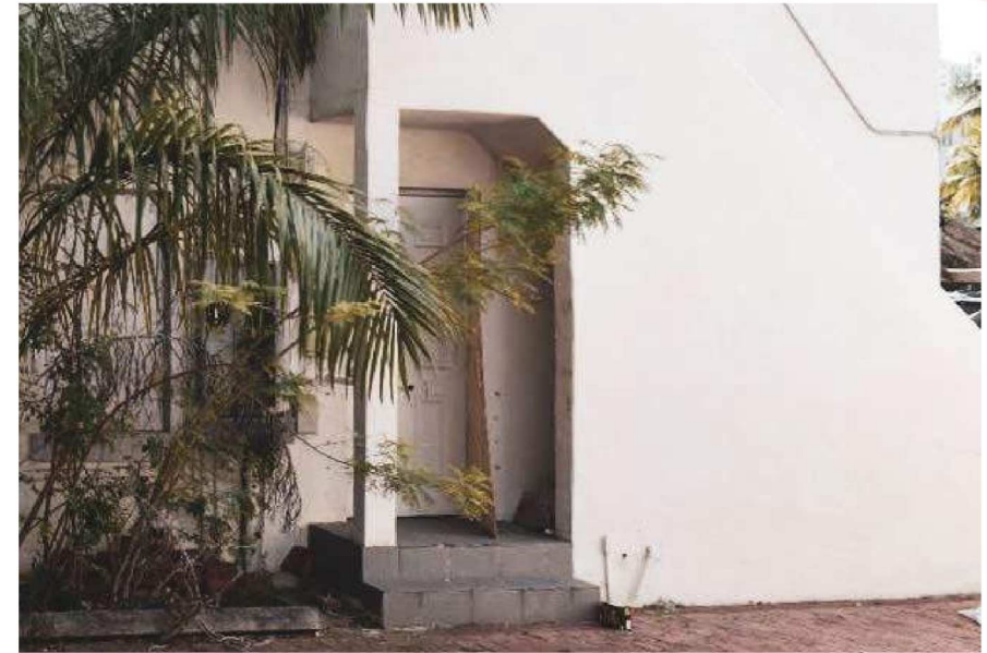
1st Level Detail NON-ORIGINAL DOOR OPENING
