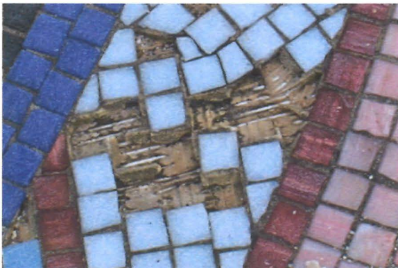
Detail of visible fiberglass mesh
