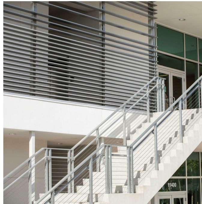
HORIZONTAL ALUMINUM LOUVERS FOR MAIN ENTRANCE
