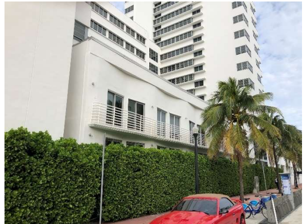
Fig. 59. Detail of accordion wall at south elevation, December 2020.
