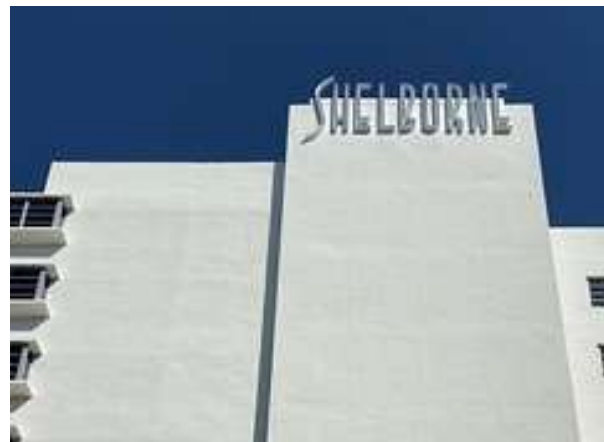
Fig. 63. Signage at top of west tower, August 2020.
