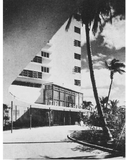
Fig. 32. Curved canopy and drive leading to lobby, 1941. (Architectural Record, July 1941, p. 42 )
