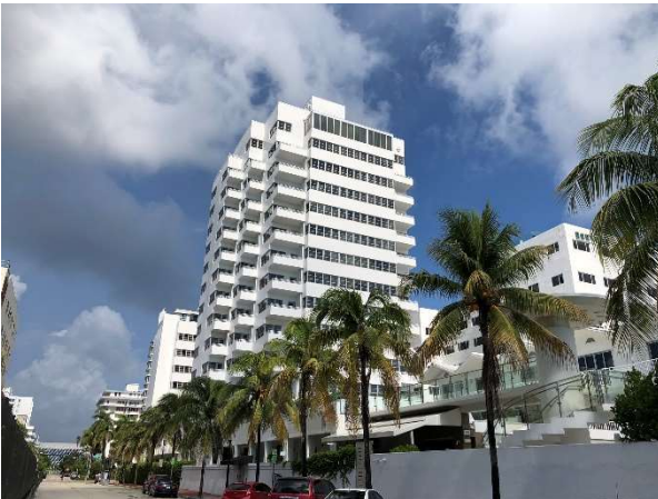
Fig. 58. South elevation, August 2020.
