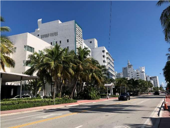
Fig. 9. East side of Collins Avenue north of the Shelborne, looking south, August 2020.
