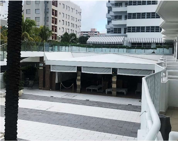
Fig. 71. Patio and upper level terrace, August 2020. (Grace Dillon, Claro Development)
