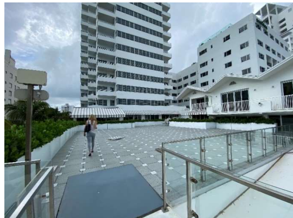
Fig. 74. Upper level terrace, August 2020. (Grace Dillon, Claro Development)
