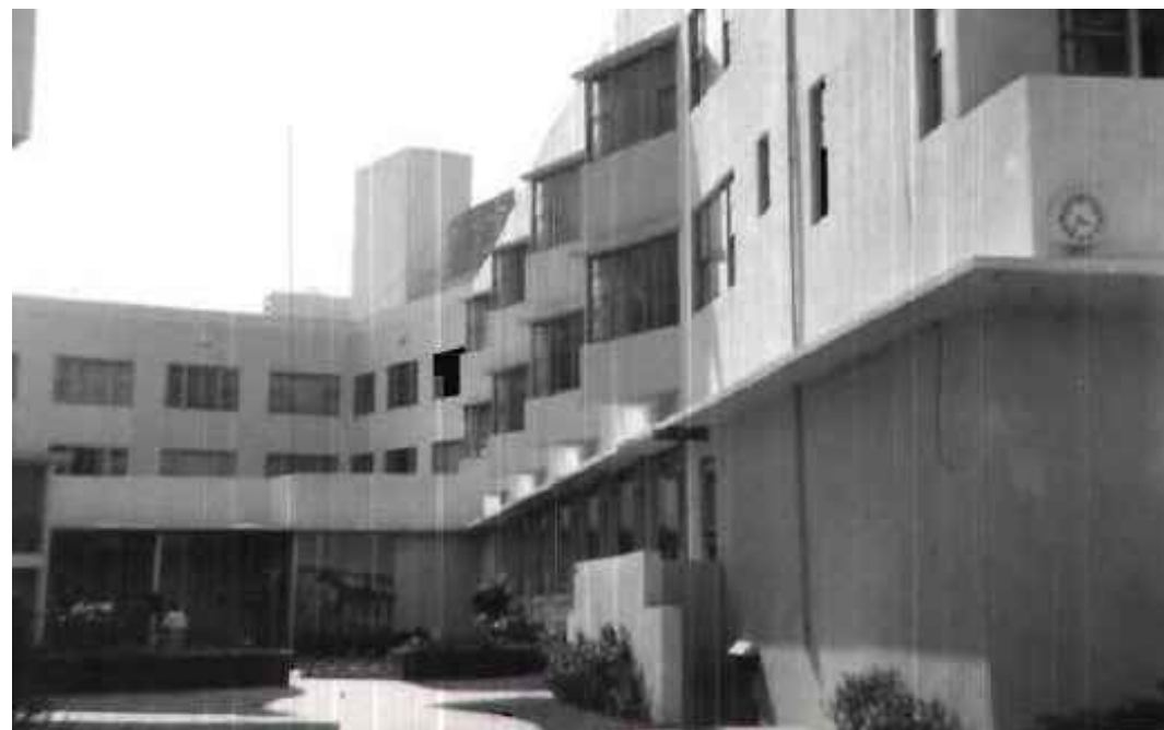
VIEW OF COURTHYARD AREA, c. 1951
