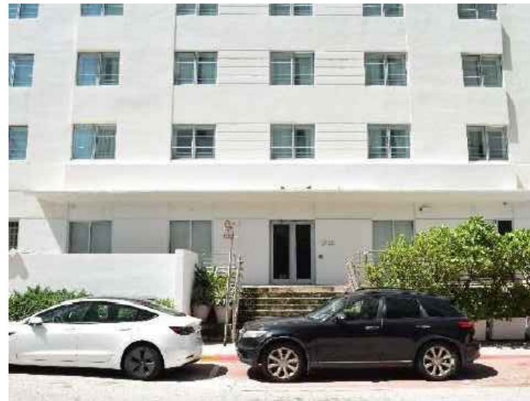
DETAIL OF BASE AT NORTH ELEVATION ENTRANCE
