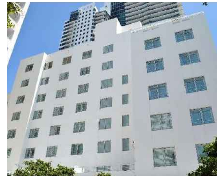
DETAIL OF FENESTRATION PATTERN AT SOUTH ELEVATION
