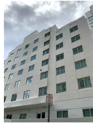
VIEW OF NORTH ELEVATION OF FORMER CROMWELL
