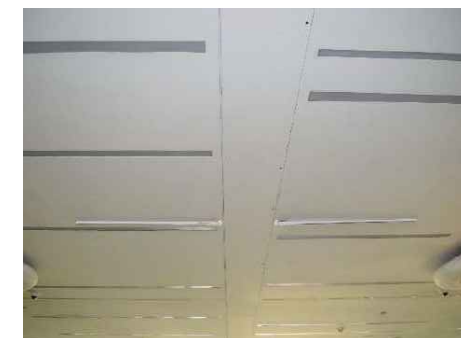
DETAIL OF CELING AT LOBBY
