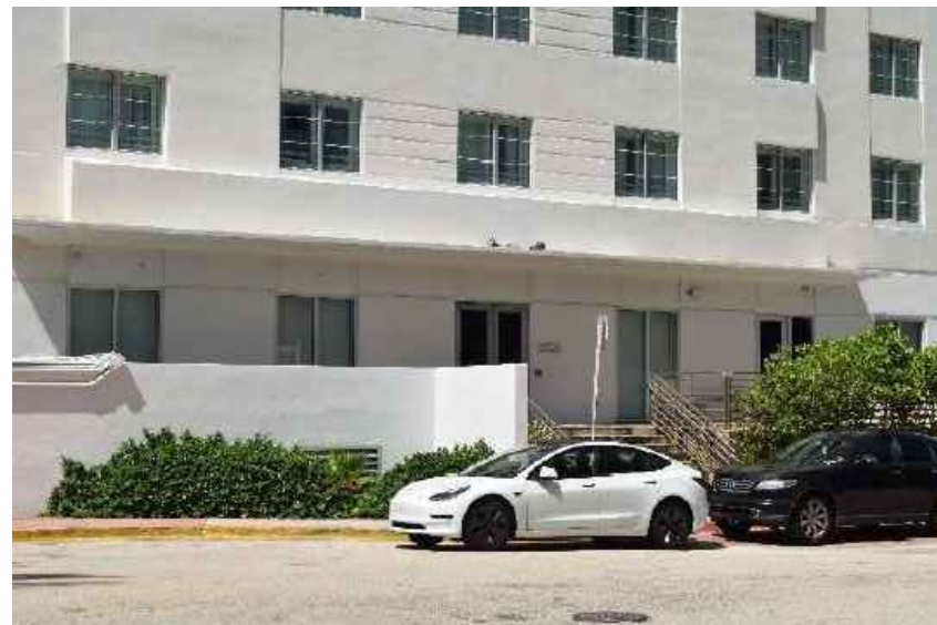
DETAIL OF FRONT WALL AT NORTH ELEVATION
