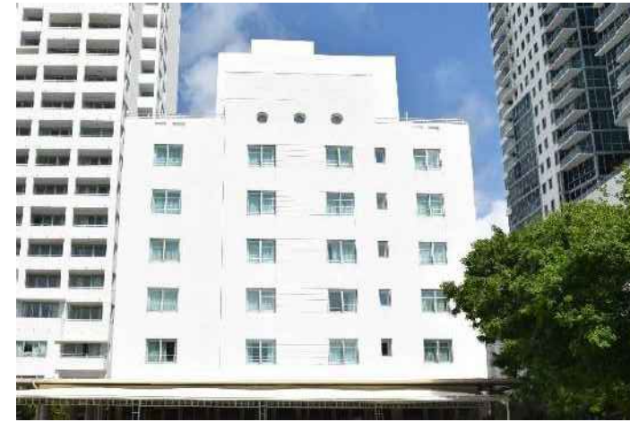
DETAIL OF FENESTRATION PATTERN AT EAST ELEVATION
