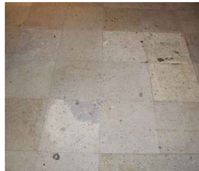
DETAIL OF FLOORING IN LOBBY
