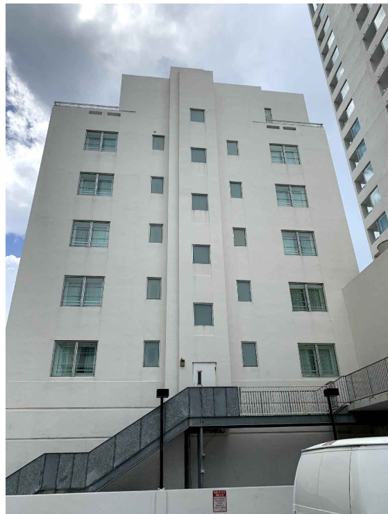
DETAIL OF FENESTRATION PATTERN AT WEST ELEVATION
