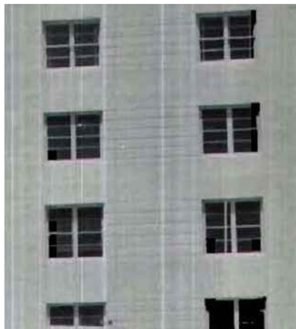
DETAIL OF ORIGINAL WINDOW MUNTING PATTERN, c. 1951
