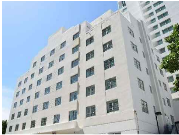
VIEW OF NORTH ELEVATION OF FORMER CROMWELL
