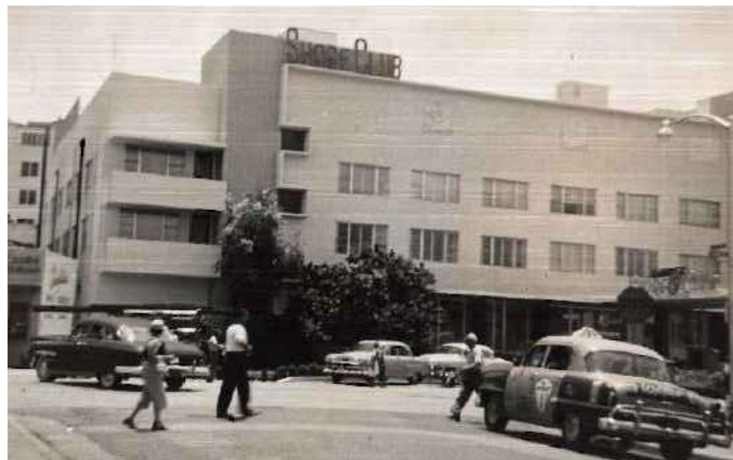
VIEW OF NORTH END OF FRONT (WEST ELEVATION) OF SHORE CLUB, c. 1951
