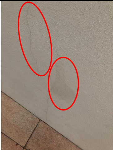
Linear Crack on the wall
