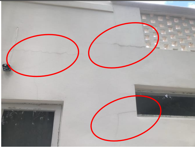
Linear Crack on the wall
