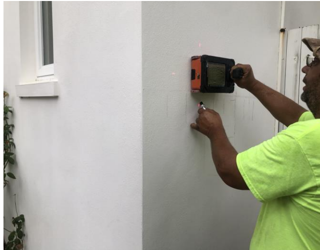
Image 1. GPR on the wall.
