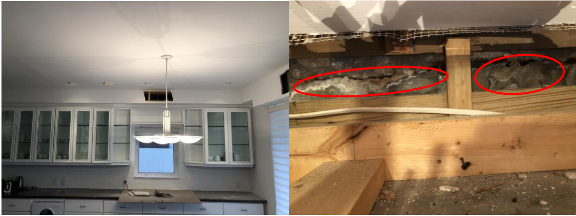
Image 2. Remove drywall to verify the situation of the concrete tie beam
