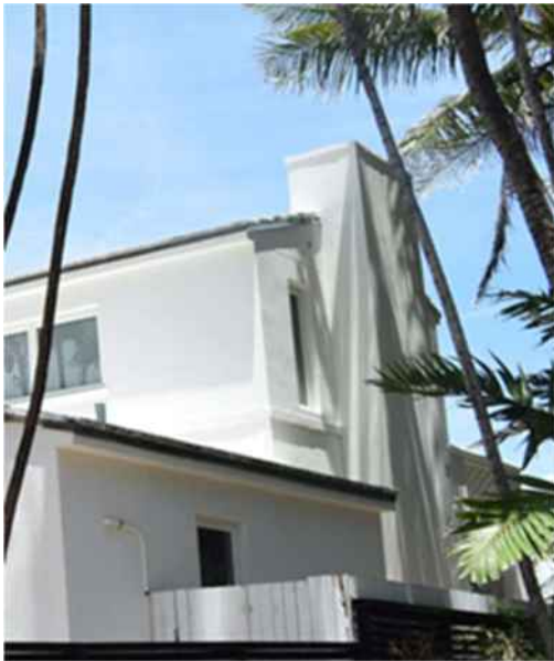
Fig. 78. View of south elevation of southern wing, May 2021.
