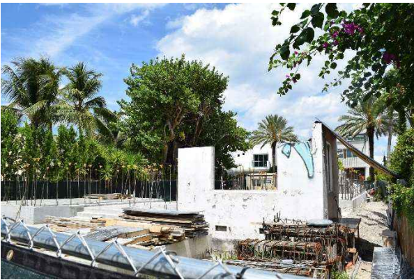
Fig. 31. 7711 Collins Avenue (under construction 2021), May 2021.
