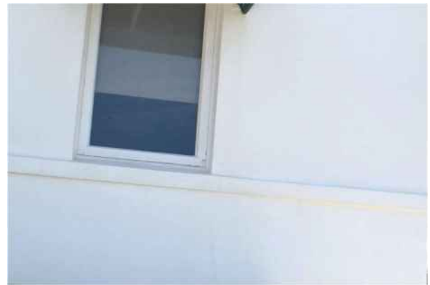
Fig. 83. Detail of belt course below second story windows, May 2021.
