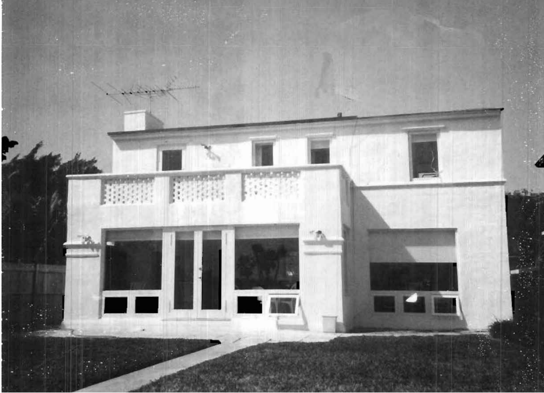
Fig. 40. View of east elevation showing enclosed porch, February 1995. (Office of the Property Appraiser, Miami-Dade County)
