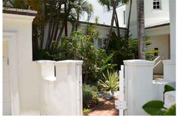
Fig. 77. View of north wing between garage and two-story portion of residence, May 2021.
