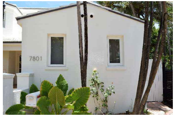
Fig. 75. View of west elevation of southern wing, May 2021.
