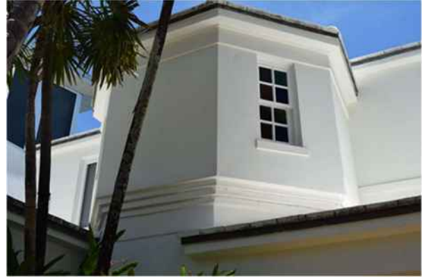
Fig. 73. Detail of octagonal stair tower with cornice and corbelled detailing, May 2021.
