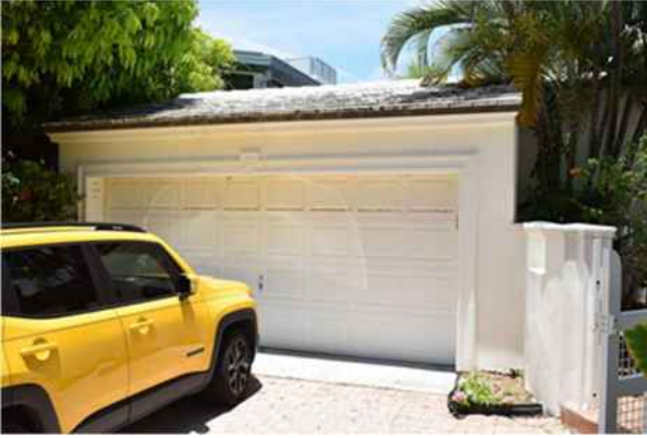
Fig. 76. View of garage with wood molding and centered "keystone" detail, May 2021.
