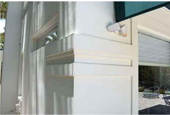
Fig. 82. Detail of paired horizontal molding, May 2021.
