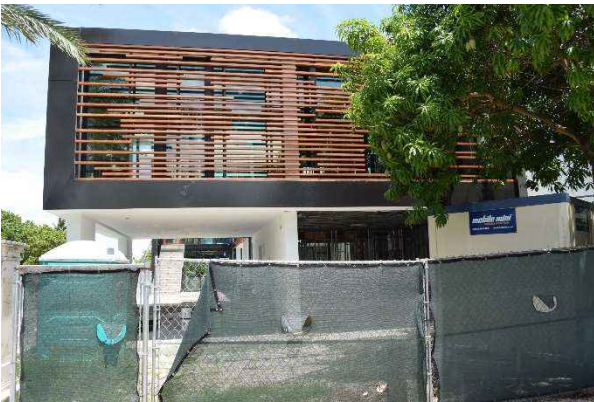
Fig. 21. 7845 Atlantic Way (under construction 2021), May 2021.
