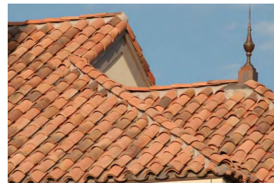
CLAY BARREL TILE ROOF
