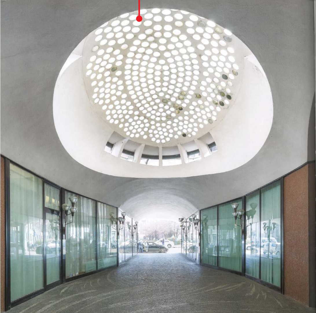
Ceiling design by Luigi Caccia Dominioni, 1957-61, Entryways of Milan
