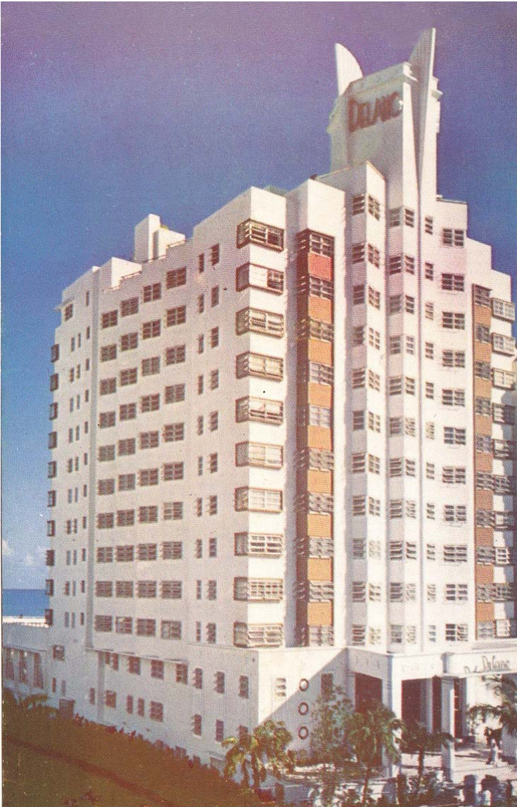
Delano facade with painted boxed windows and window frames
