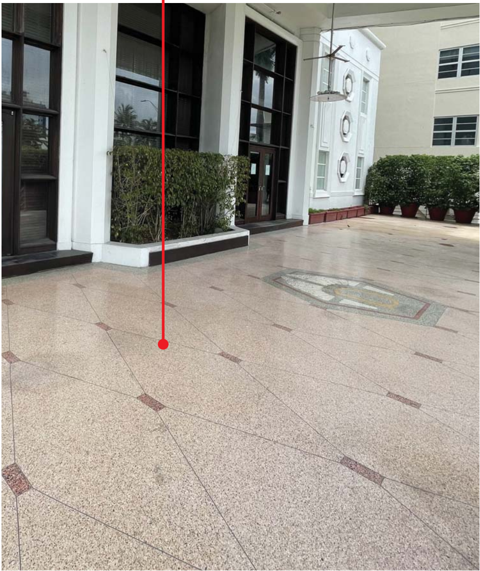
Existing terrazzo at Delano entry
