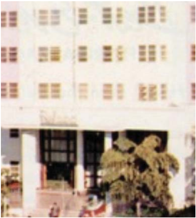
Original mullions at entry doors
