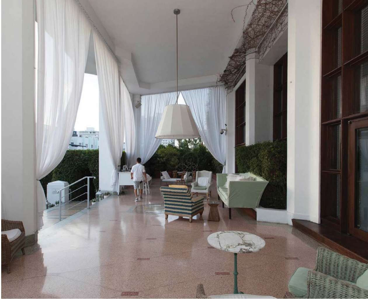
Existing terrazzo flooring at entry terrace
