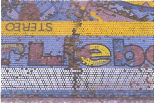
Detail of missing tesserae both spread out and in a linear pattern as seen in the center of the image.
