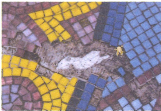
Detail of the bedding mortar and underlying fiberglass and mesh.
