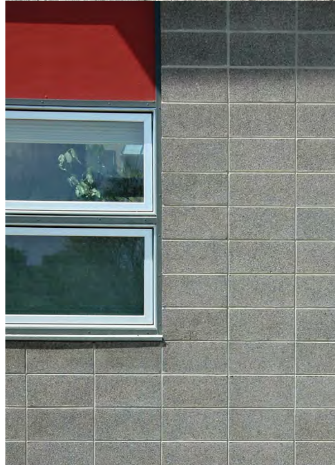
GROUND FACE STACKED BOND MASONRY VENEER ECHELON TRENDSTONE, COLOR: GRAYSTONE
