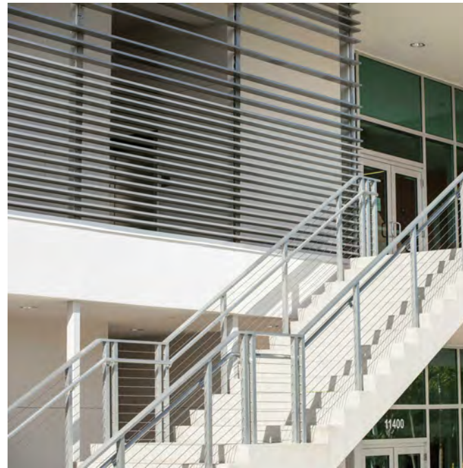
ALUMINUM HORIZONTAL SCREEN FOR STAIR ENCLOSURE
