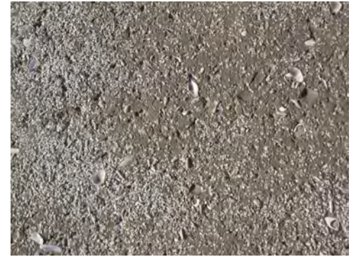
SEASHELL CONCRETE FOR APPARATUS BAY RAMPS
