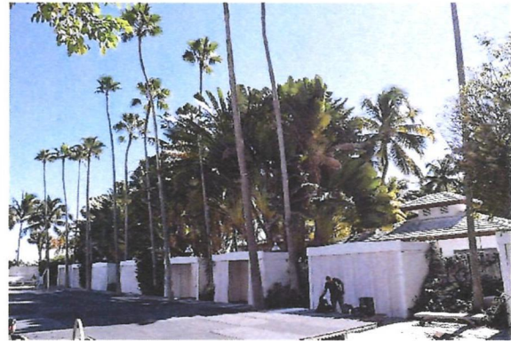
Figure 19. One-story cabanas south of pool, December 2021. (Heritage Architectural Associates)
