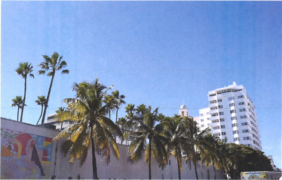
Figure 39. View of (l-r) Ritz-Carlton, Sagamore, National, Delano and SLS (Ritz Plaza) from 17 th Street, December 2021.
