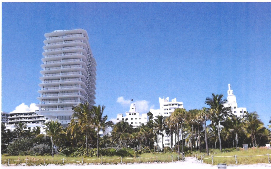
Figure 34. Rendering showing proposed tower in relation to area hotels, October 2021. (Heritage Architectural Associates with K4 Architecture)
