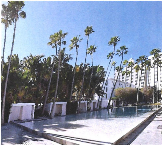
Figure 41. View of pool area at Delano Hotel, looking southwest, December 2021. (Heritage Architectural Associates)
