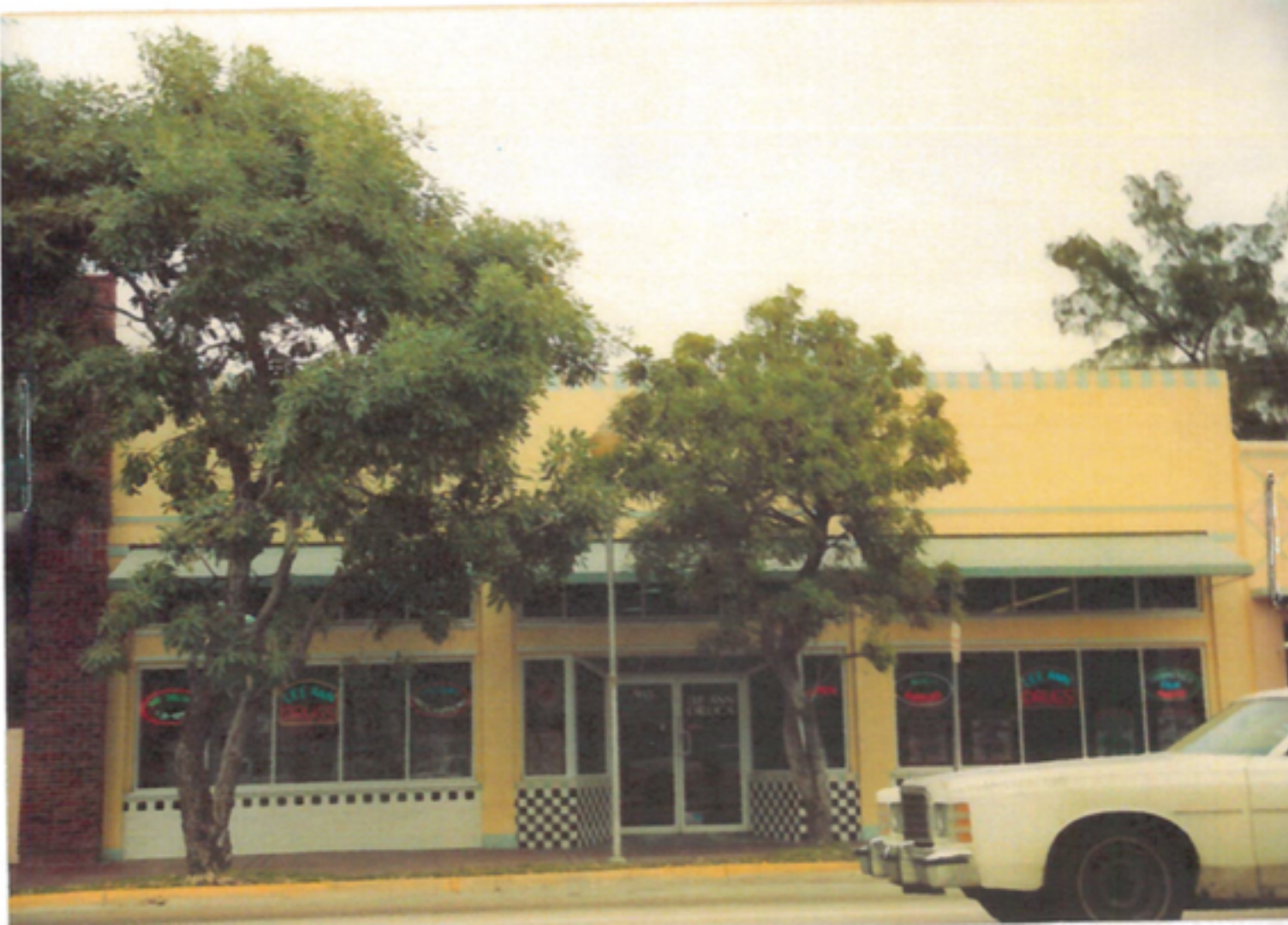
Above 1989 PHOTOGRAPH from the CITY OF MIAMI BEACH PLANNING DEPARTMENT's HISTORIC PROPERTIES DATABASE Note that this photo shows the double-crenelated parapet top pre-installation of the non-historic wave neon lights. See 2015 detail photographs on following page.
