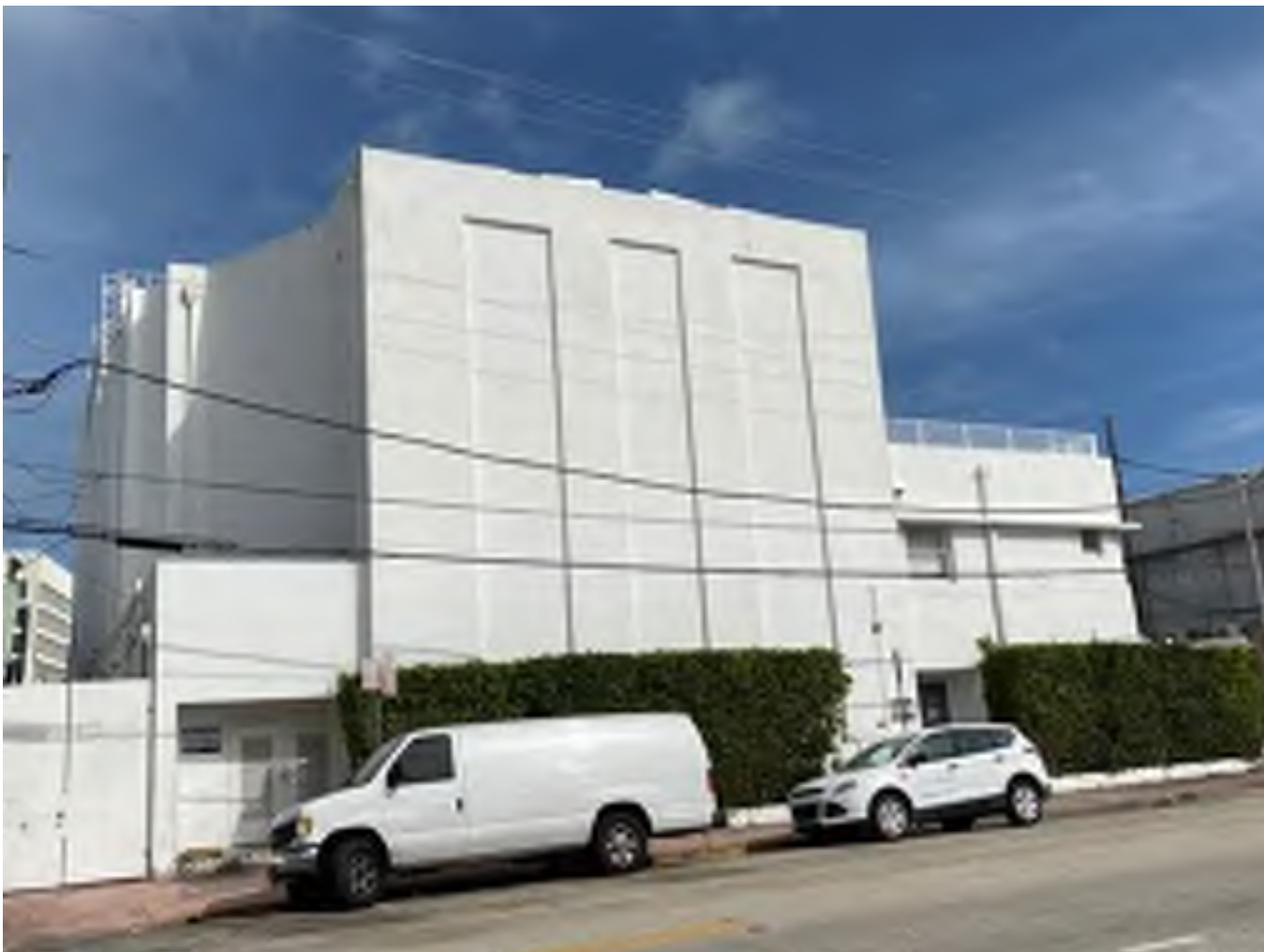
ABOVE: LOOKING NW FROM EUCLID AVENUE WITH SOUTH ELEVATION AT RIGHT AND WEST ELEVATION AT LEFT. (23)
