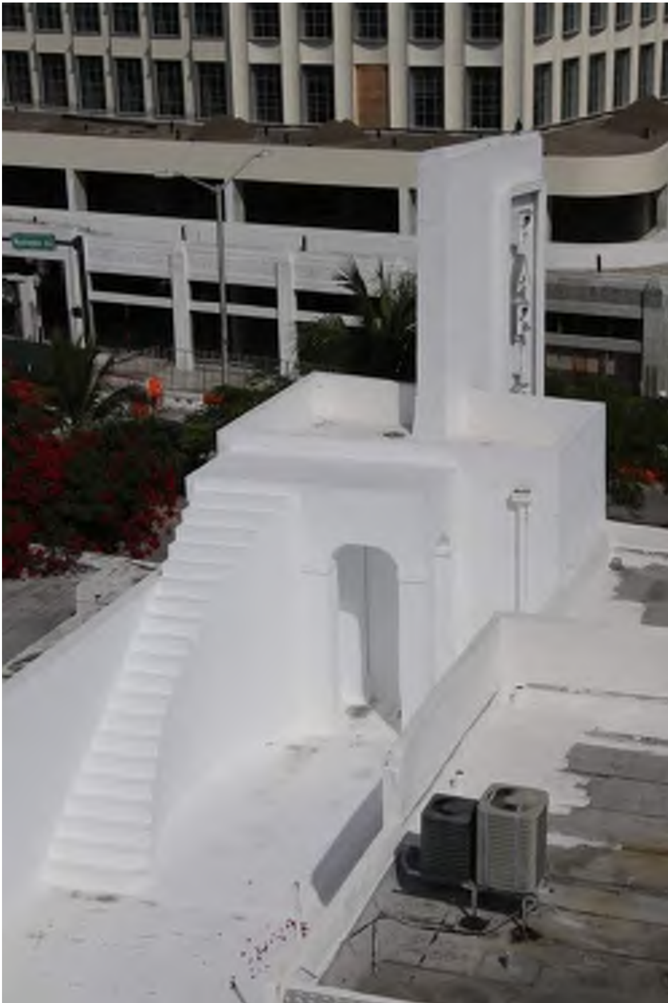
ONE OF THE ROOFTOP STRUCTURES FOR PHOTOSHOOTS. (23)
