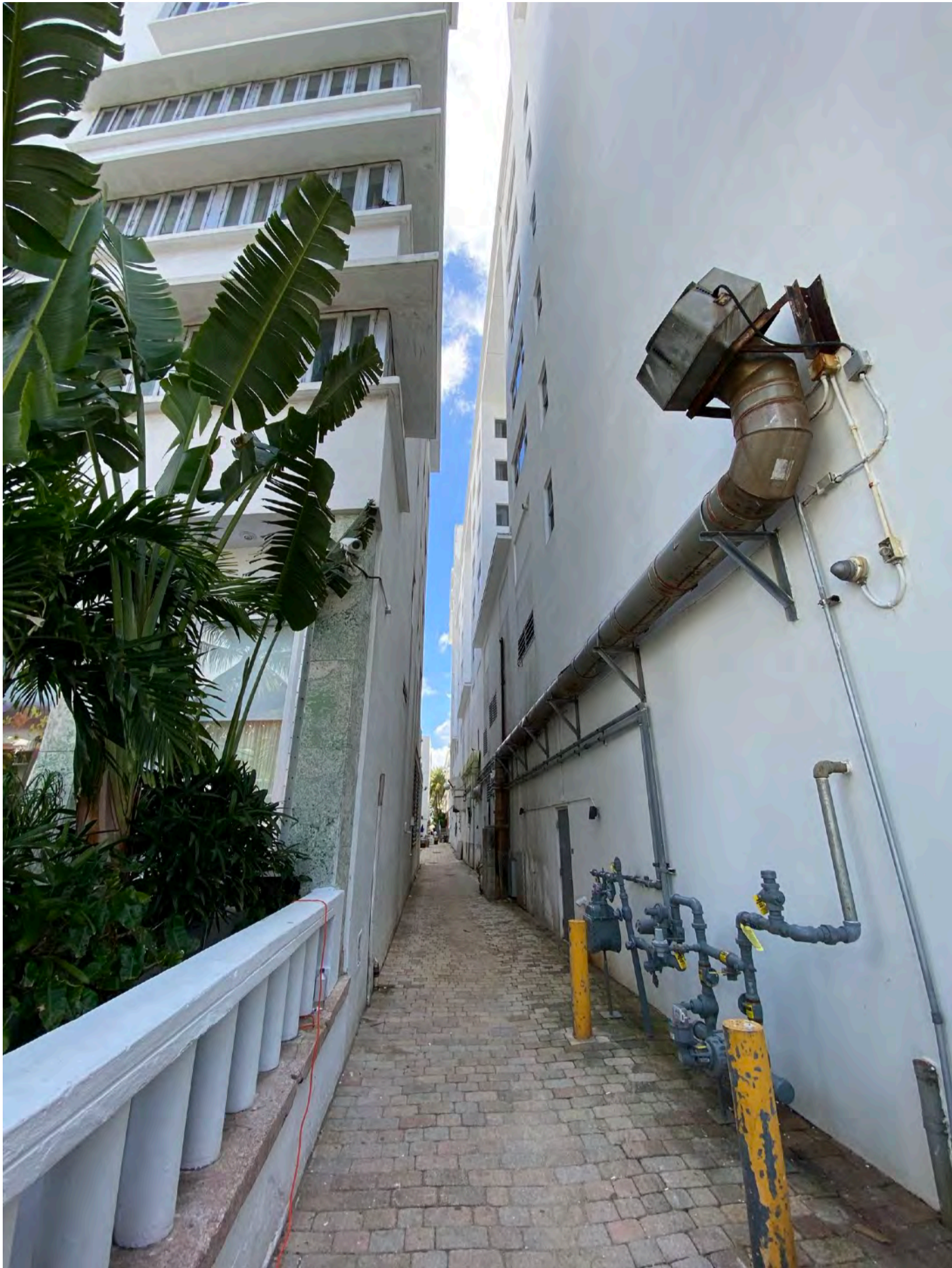
The approximately 10'-0" wide service alley between the Sagamore Hotel at left and the Ritz Carlton DiLido Hotel at right. (24)
