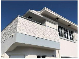
Fig. 39. Detail of overhanging upper walkway and stone veneer, March 2021.
