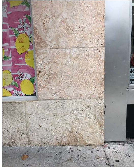
Fig. 44. Detail of granite cladding, June 2021.
