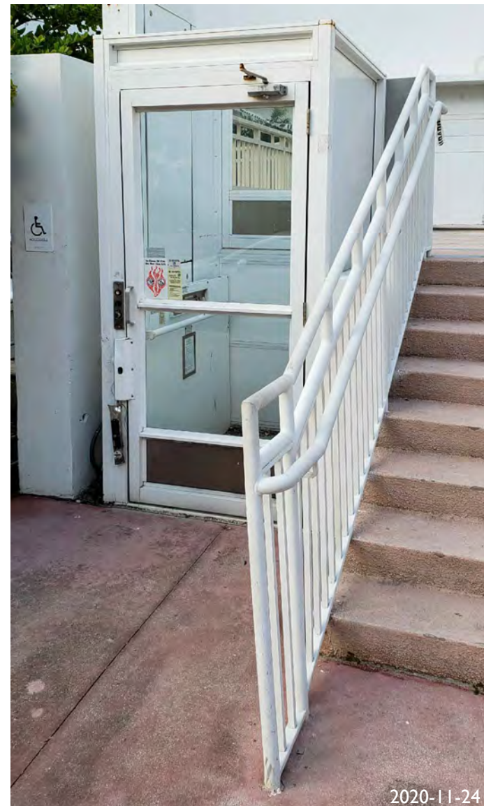
13. VIEW FACING ADA LIFT ON OCEAN STEPS
