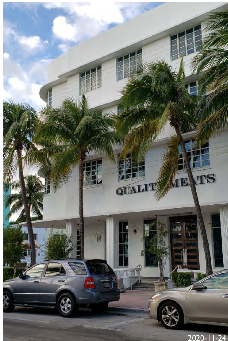
12. VIEW OF BANCROFT BUILDING FACING NW
