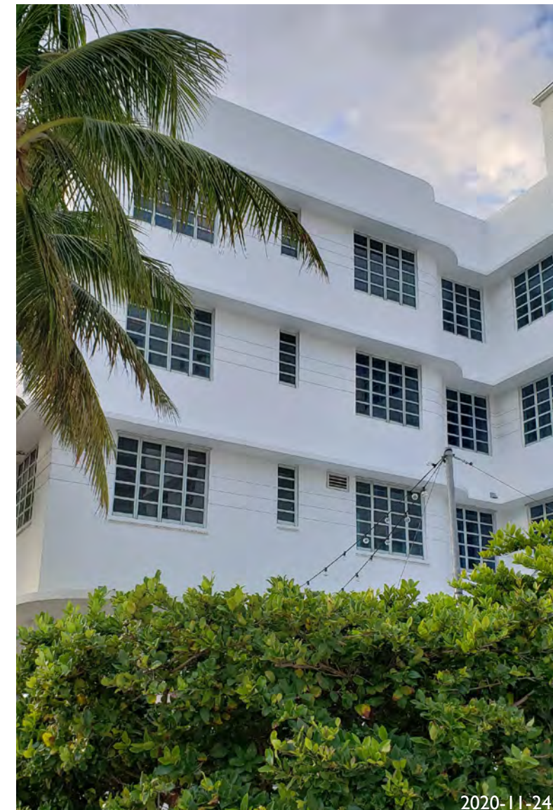
14. VIEW OF BANCROFT BUILDING FACING NW
