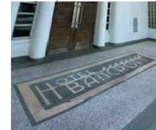
EXISTING ENTRANCE FLOOR MEDALLION TO BE PRESERVED
