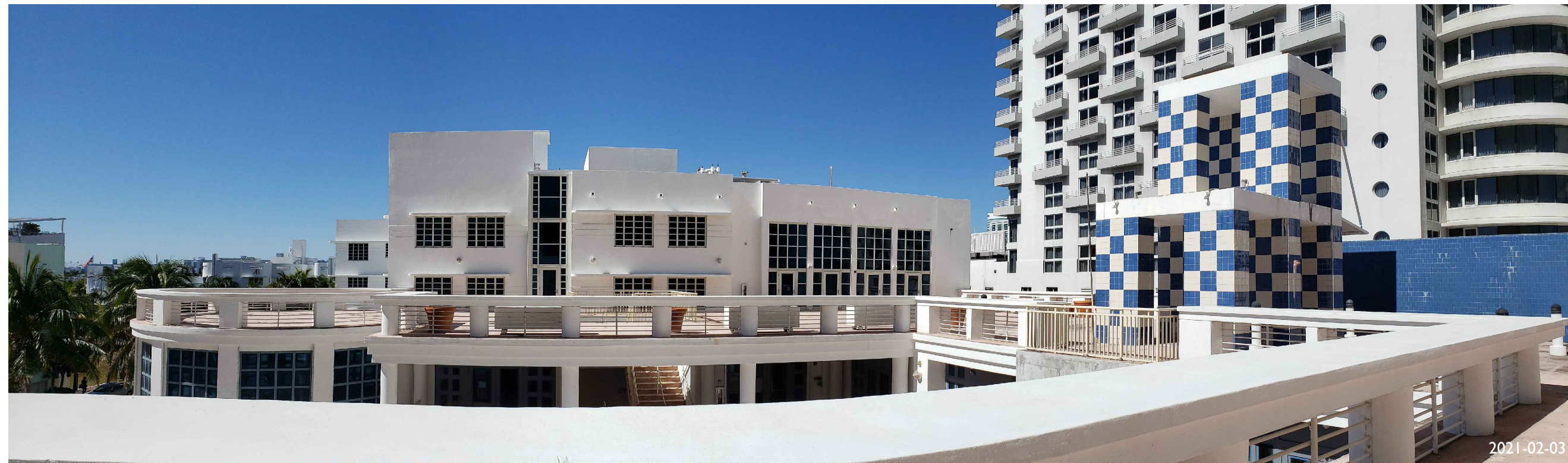
97. 3RD FLOOR TERRACE
