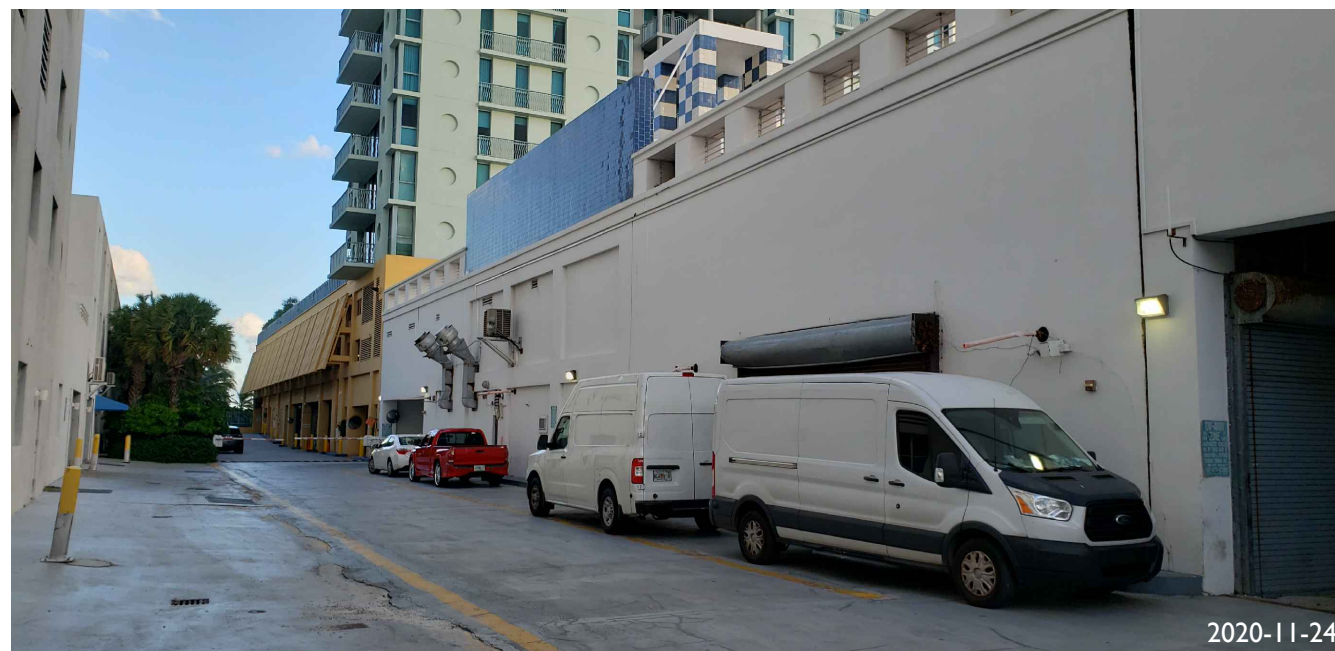
53. VIEW OF LOADING AREA, ALLEY FACING SE
