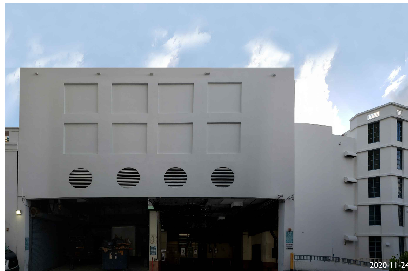
54. VIEW OF LOADING AREA, ALLEY FACING SOUTH
