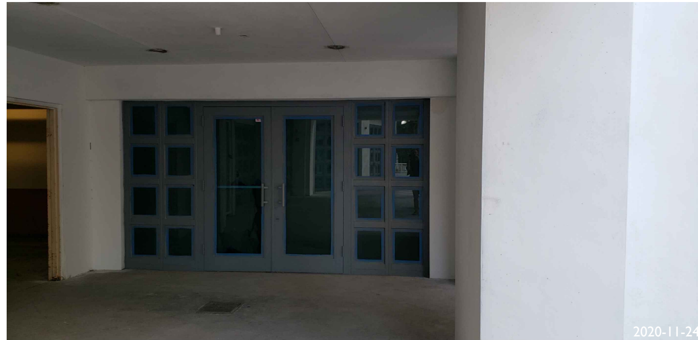
47. VIEW OF OCEAN STEPS COURTYARD
