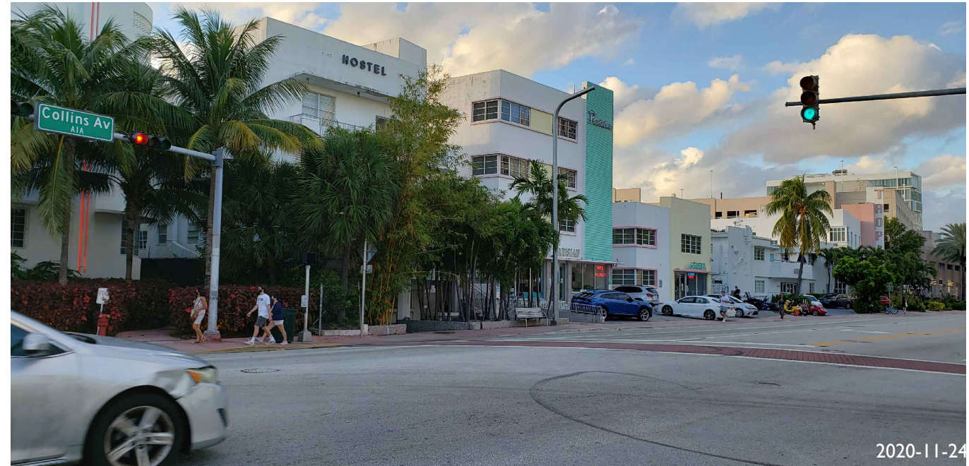
60. VIEW OF HOTELS, RETAIL ON COLLINS AVE FACING NW
