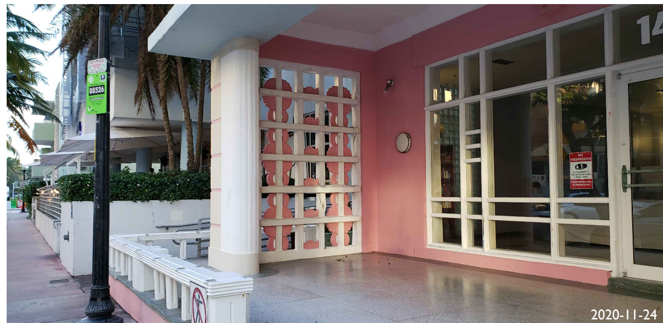
73. VIEW OF DRAKE BUILDING'S LOBBY (1460 OCEAN DR)
