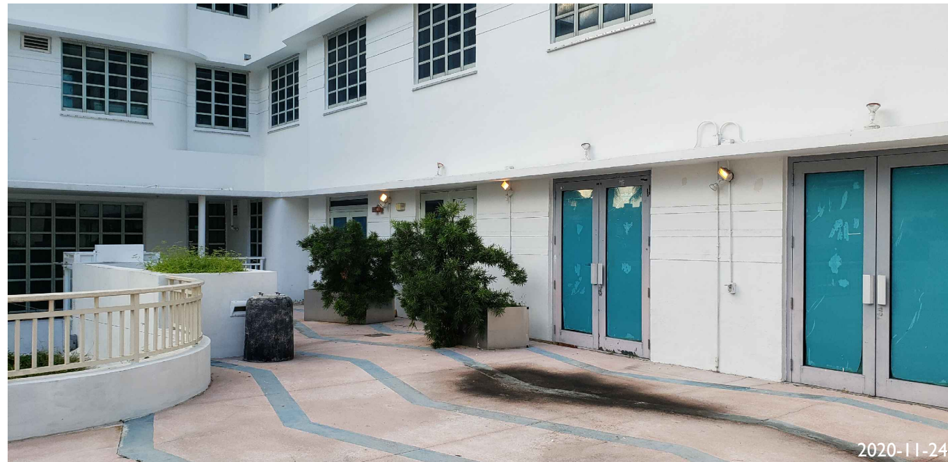
19. VIEW OF BANCROFT BUILDING FACING NW
