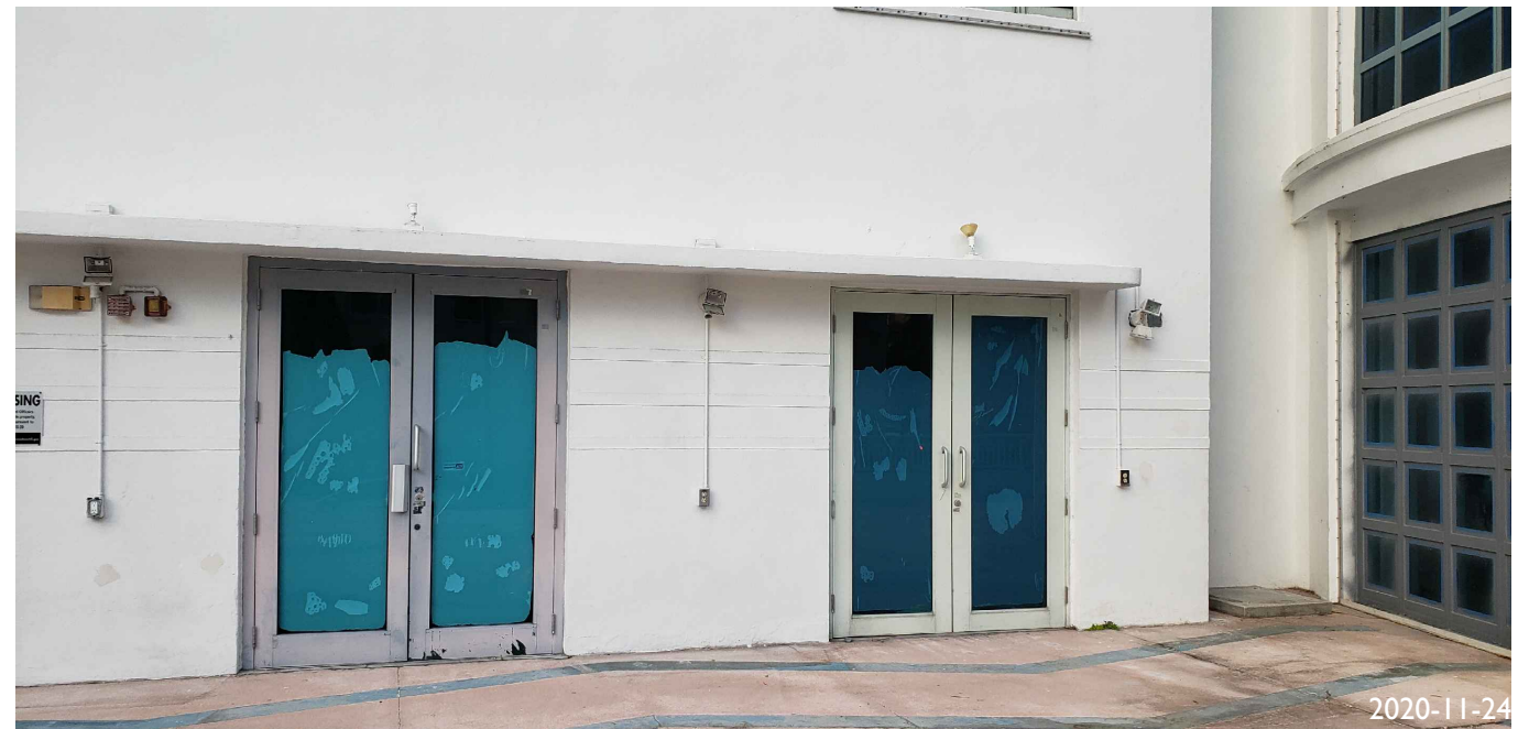
22. VIEW OF BANCROFT BUILDING FACING WEST
