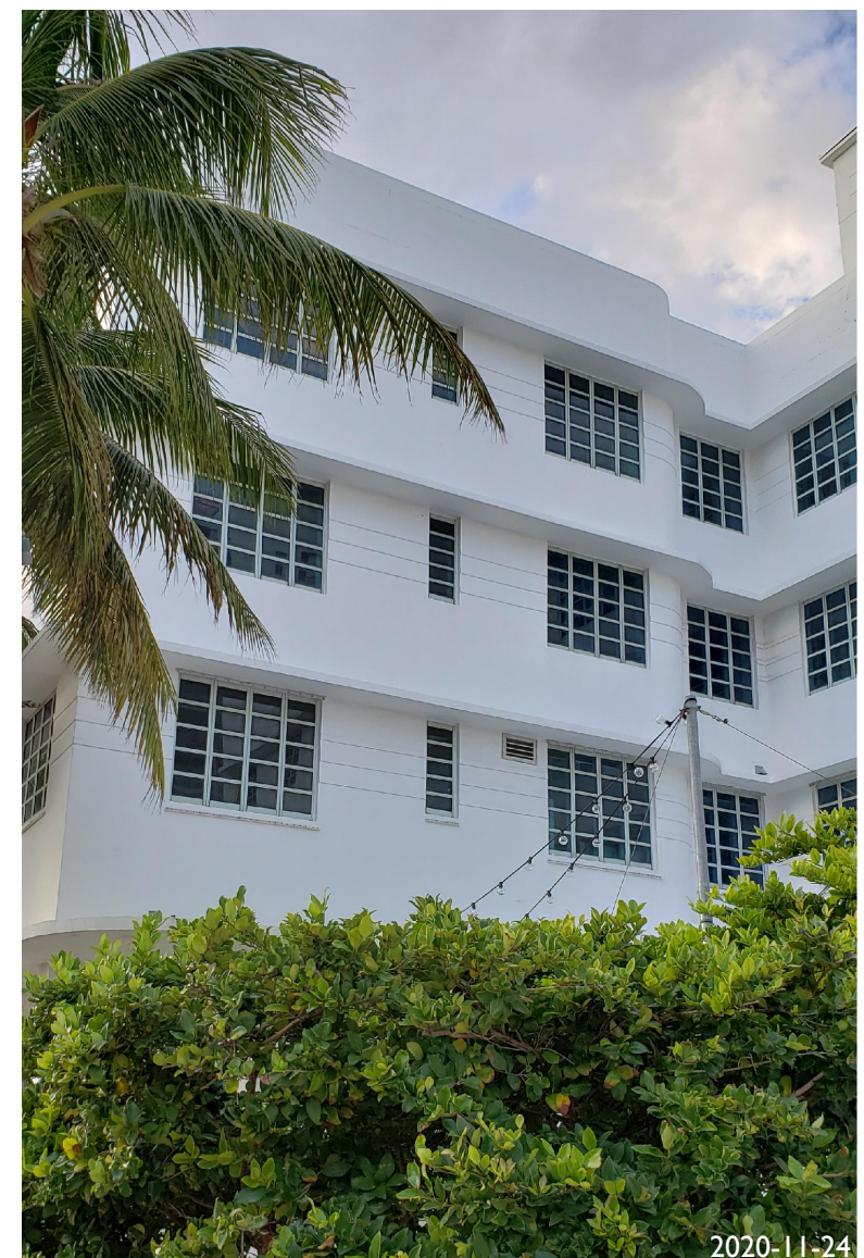
14. VIEW OF BANCROFT BUILDING FACING NW
