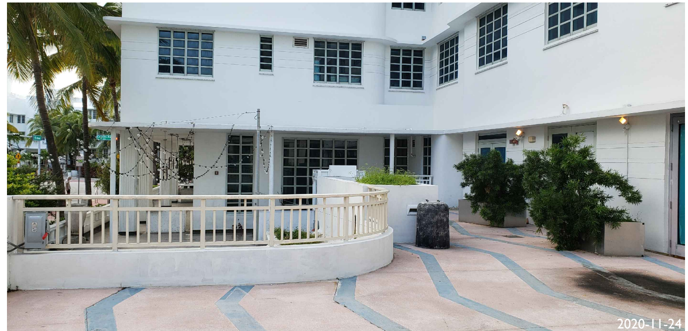
20. VIEW OF BANCROFT BUILDING FACING WEST
