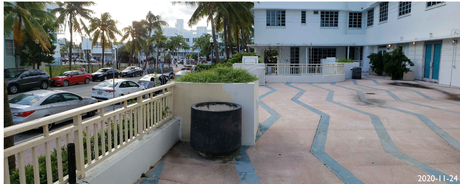
2020-11-24 30. VIEW OF BANCROFT BUILDING FACING WEST
