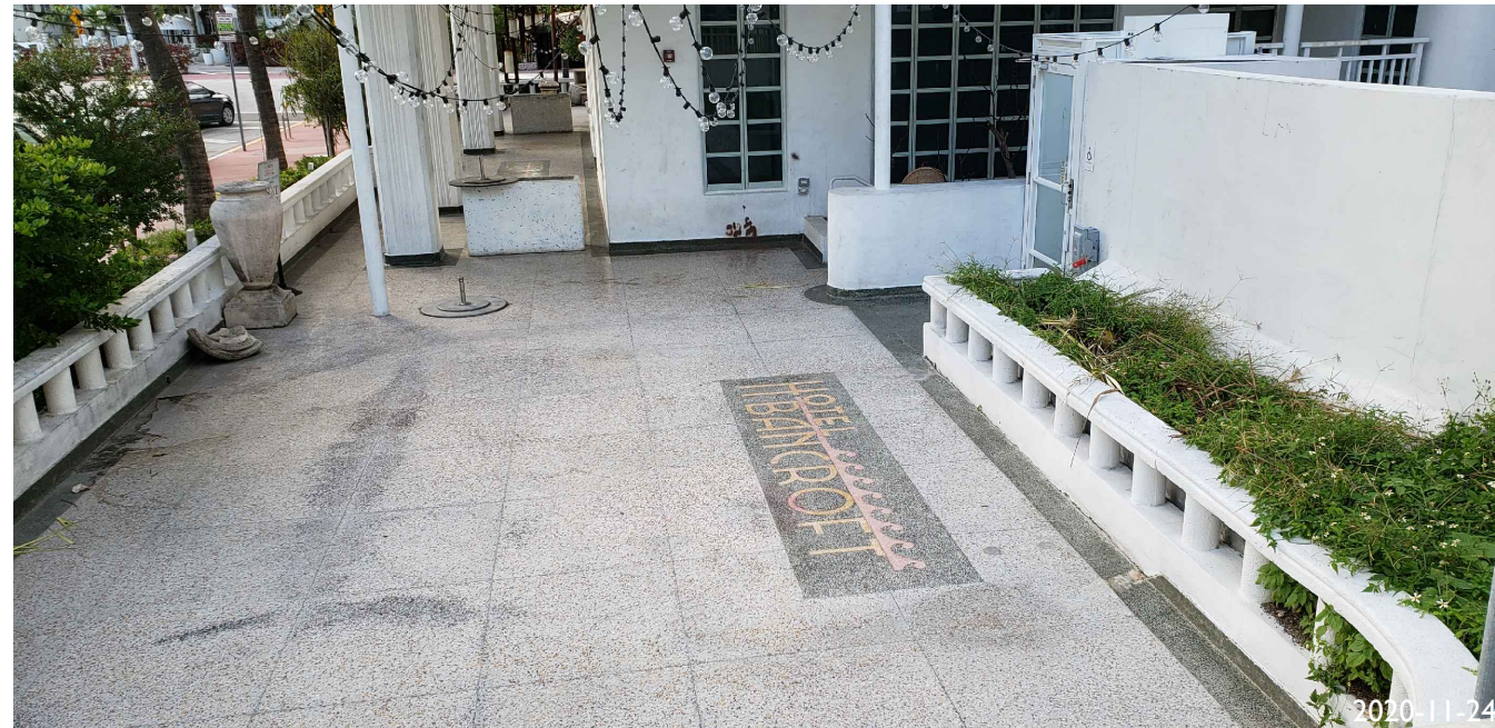
23. VIEW OF BANCROFT BUILDING FACING WEST
