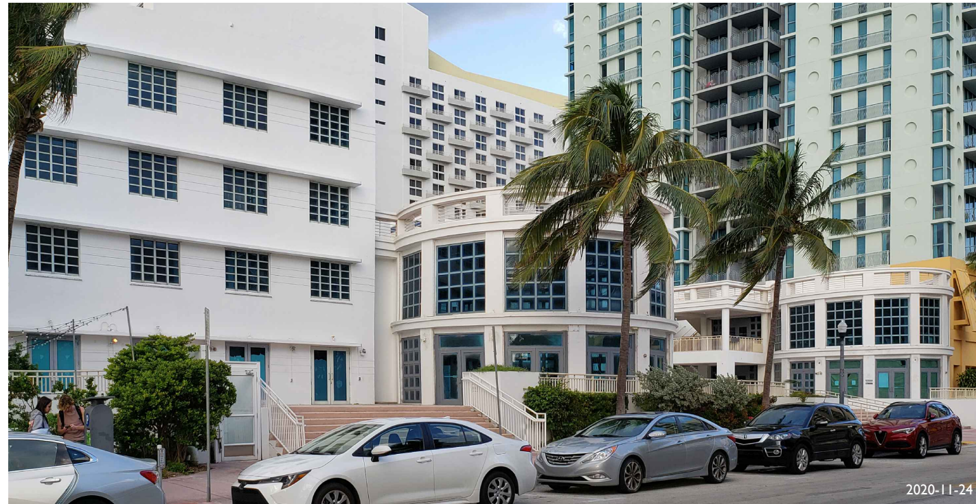
2. VIEW FACING NORTHEAST, OCEAN STEPS
