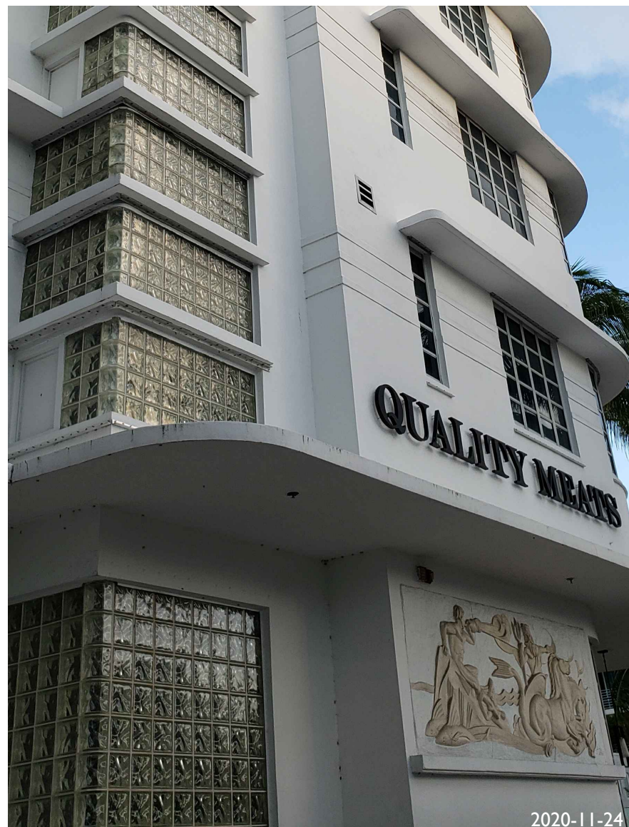
3. GLASS BLOCKS ON WEST FACADE
