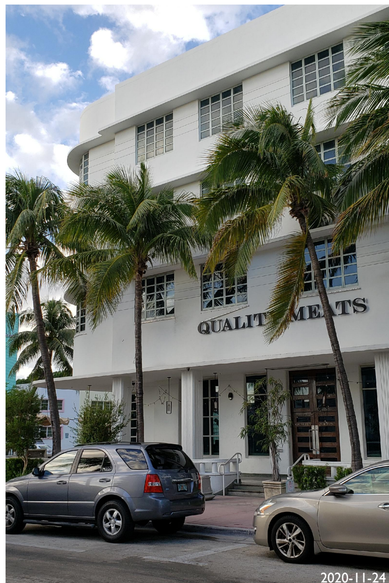
12. VIEW OF BANCROFT BUILDING FACING NW
