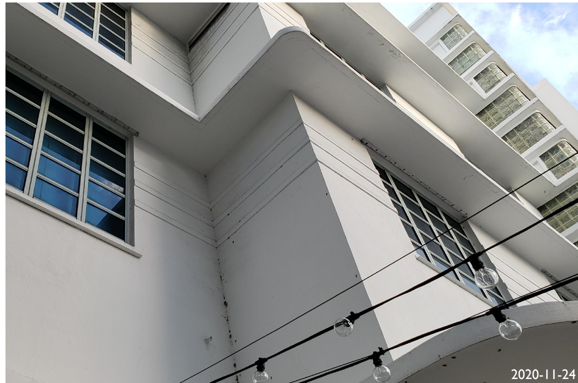
9. STRAIGHT ANGLE FACADE WITH CHAMFERED BRIS SOLEIL
