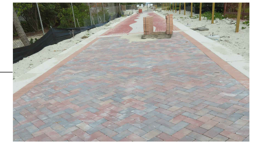
CITY OF MIAMI BEACH RECREATIONAL CORRIDOR UNDER CONSTRUCTION
