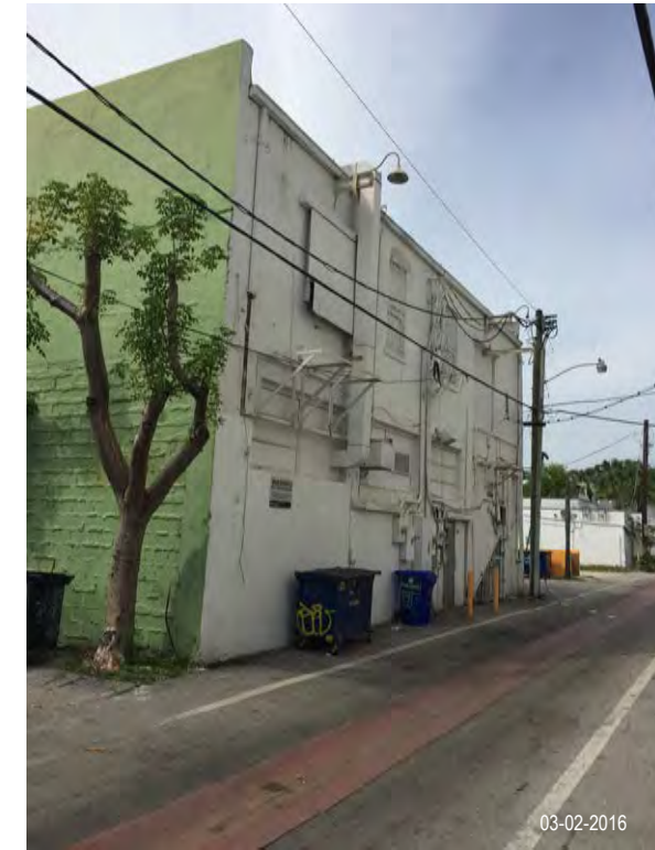
REAR ELEVATION AT COLLINS COURT: 719 WASHINGTON AVE
