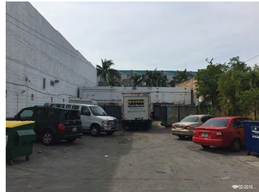
REAR ELEVATION AT COLLINS COURT: 729 WASHINGTON AVE
