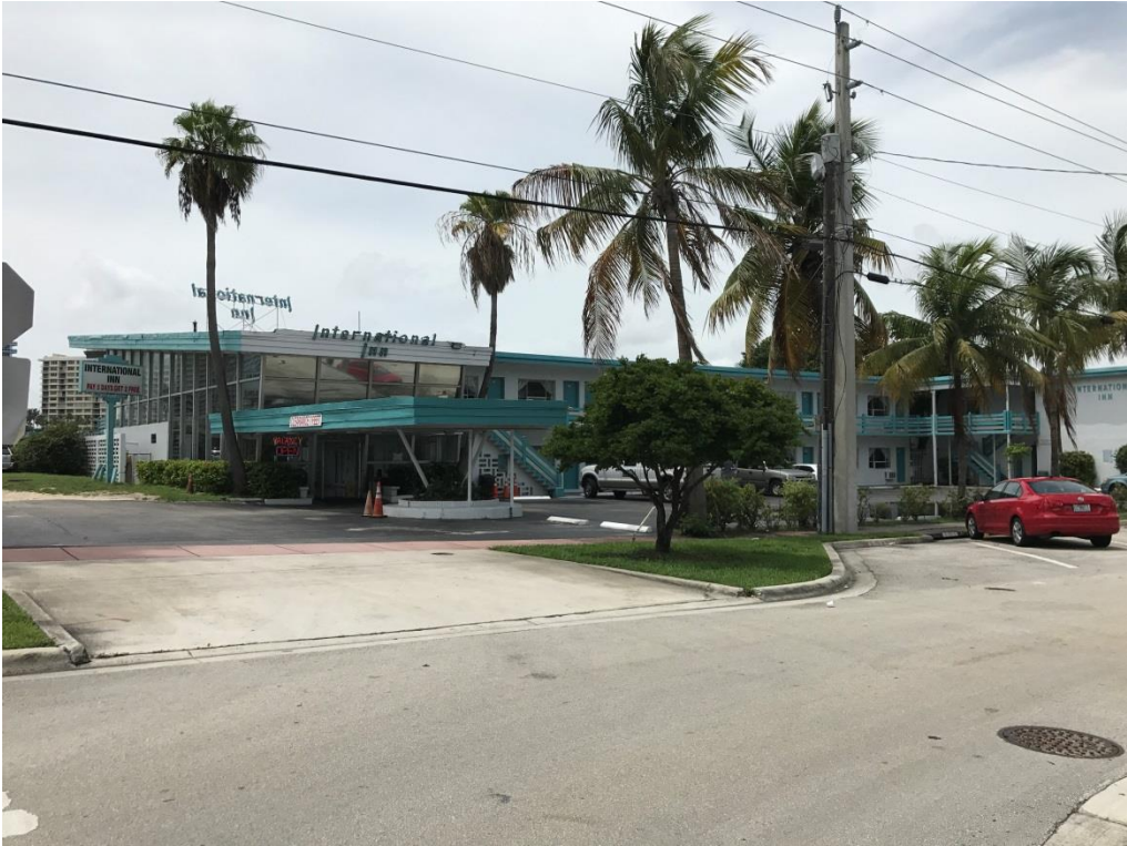
2301 Normandy Drive, view looking northwest, 2018
