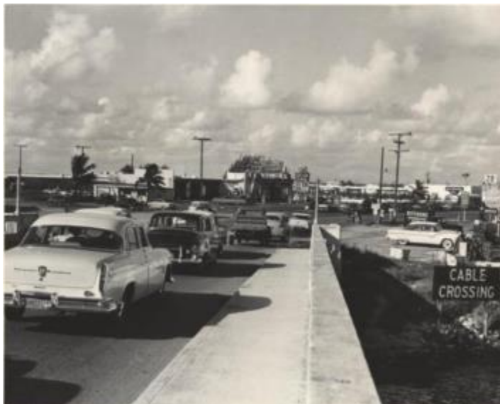
View looking west, 79 th Street Causeway, 1955
