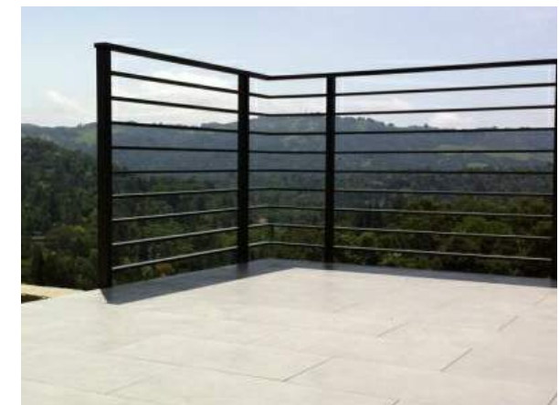
24 METAL GUARDRAIL SYSTEM W/KYNAR FINISH COMPLYING W/AAMA 2605 (IMAGE FOR VISUAL REFERENCE ONLY)
