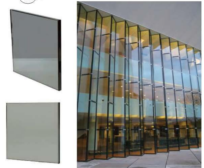
02 ALUMINUM WINDOW WALL ASSEMBLY W/KYNAR FINISH COMPLYING W/IAAMA 2605, W/ TINT LAMINATED IMPACT GLASS (IMAGES FOR VISUAL REFERENCE ONLY)
