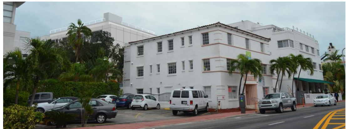
President Villa Hotel 1425 Collins Av, ground level addition
