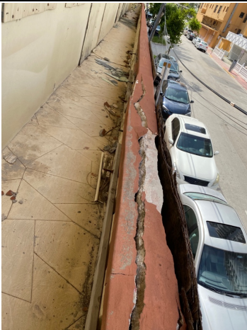
Photo 11 - South Elevation, walkway slab concrete spalling
