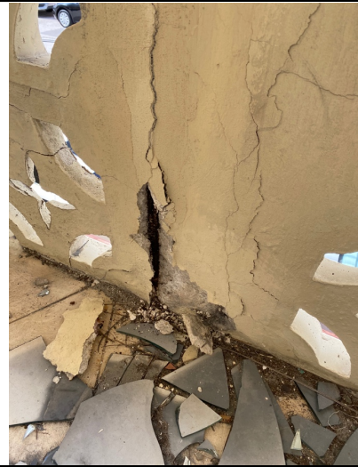
Photo 14 - Guardrail concrete spalling
