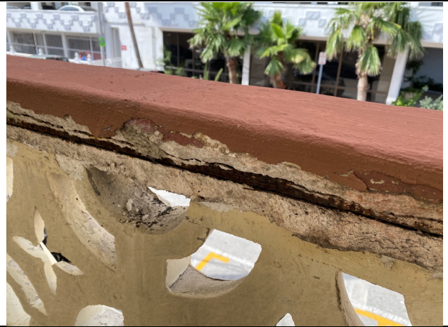
Photo 8 - Guardrail concrete spalling
