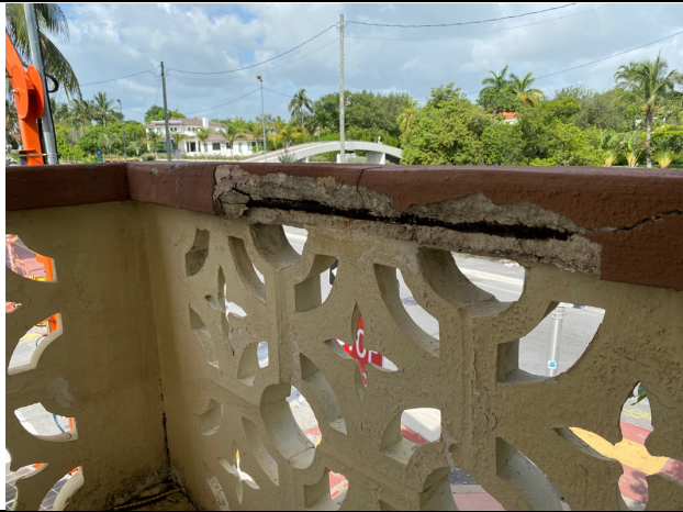
Photo 7 – Guardrail concrete spalling
