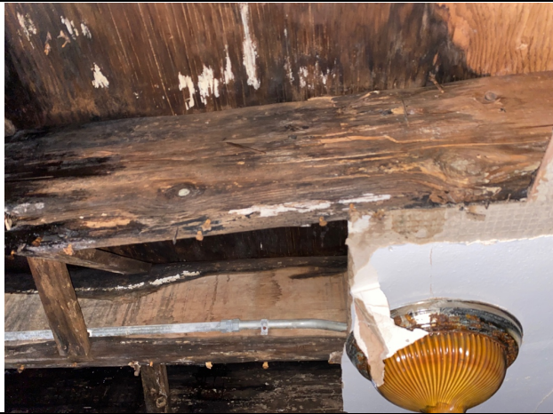
Photo 21 - 2 nd floor joist damage
