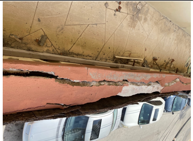
Photo 12 - South Elevation, walkway concrete spalling
