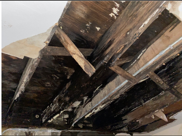
Photo 19 – 2 nd floor joist damage
