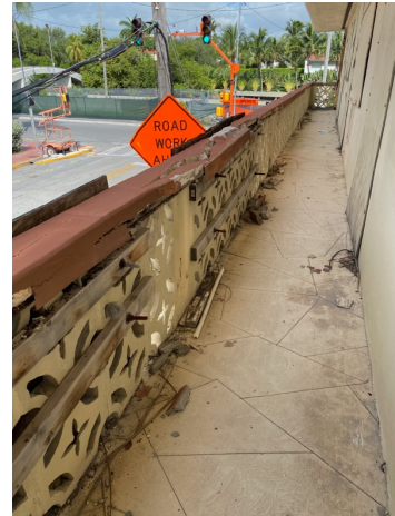
Photo 16 - Guardrail concrete spalling
