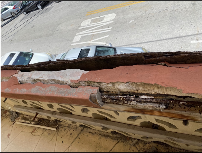
Photo 13 - Guardrail concrete spalling
