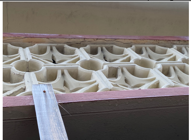
Photo 18 – South Guardrail cracking
