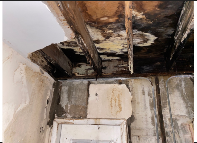
Photo 20 - 2 nd floor joist damage
