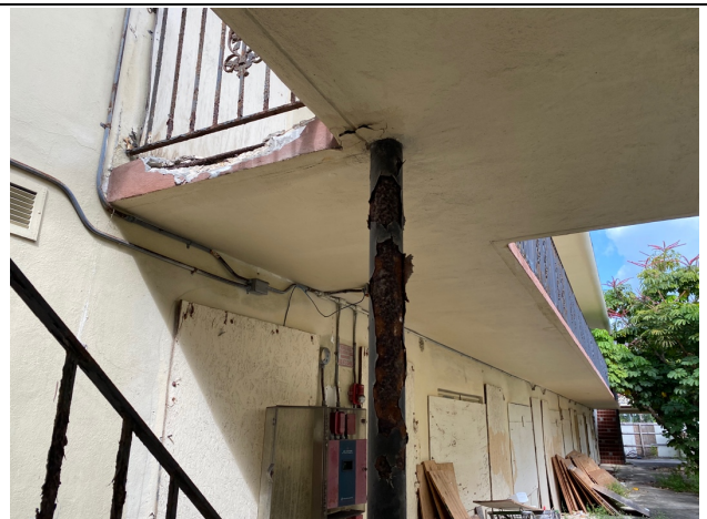
Photo 4 – Corroded Column and concrete spalling
