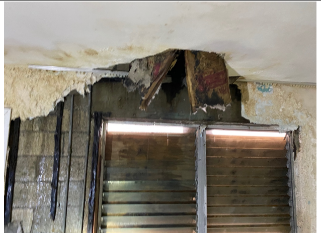
Photo 24 – Roof failure
