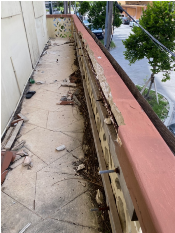
Photo 15 - Guardrail concrete spalling
