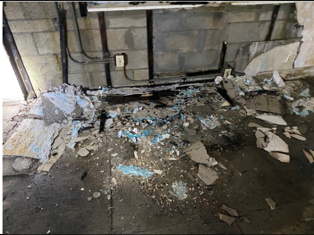
Photo 25 – Roof failure
