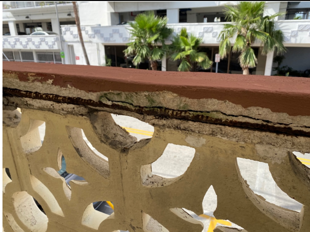
Photo 9 - Guardrail concrete spalling
