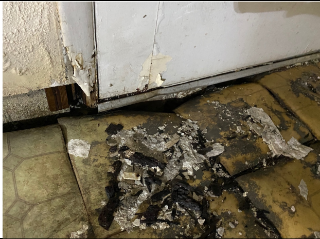
Photo 27 – Floor failure at edge of joists
