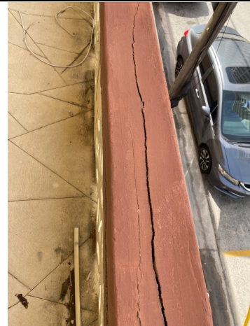
Photo 10 - Guardrail concrete cracking
