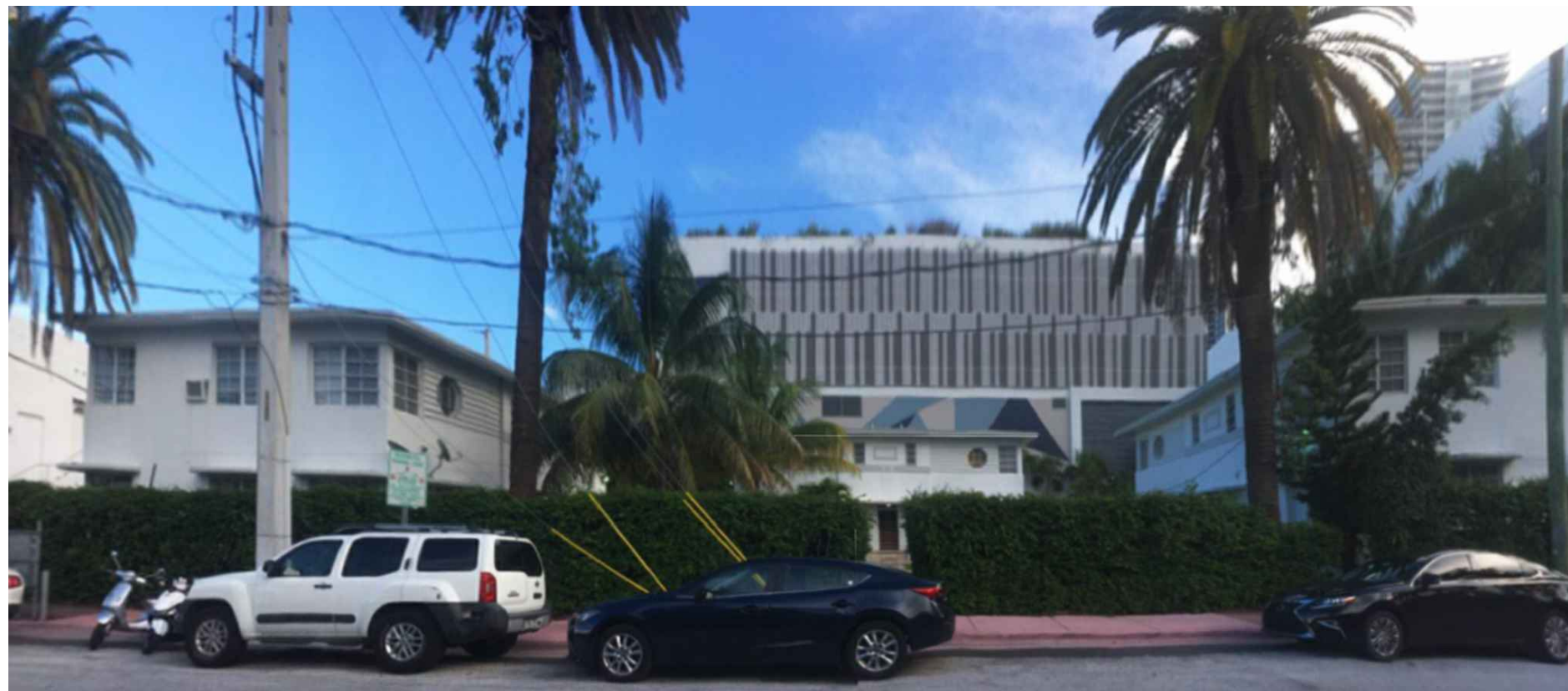
VIEW FACING SOUTH ON 6TH STREET-EXISTING
