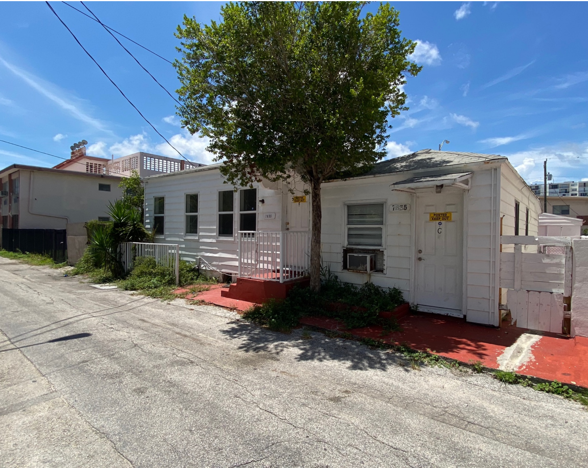
VIEW OF GUEST HOUSE ADDITION AT LEFT FROM REAR ALLEY WITH ORIGINAL CONVERTED GARAGE AT RIGHT (11)
