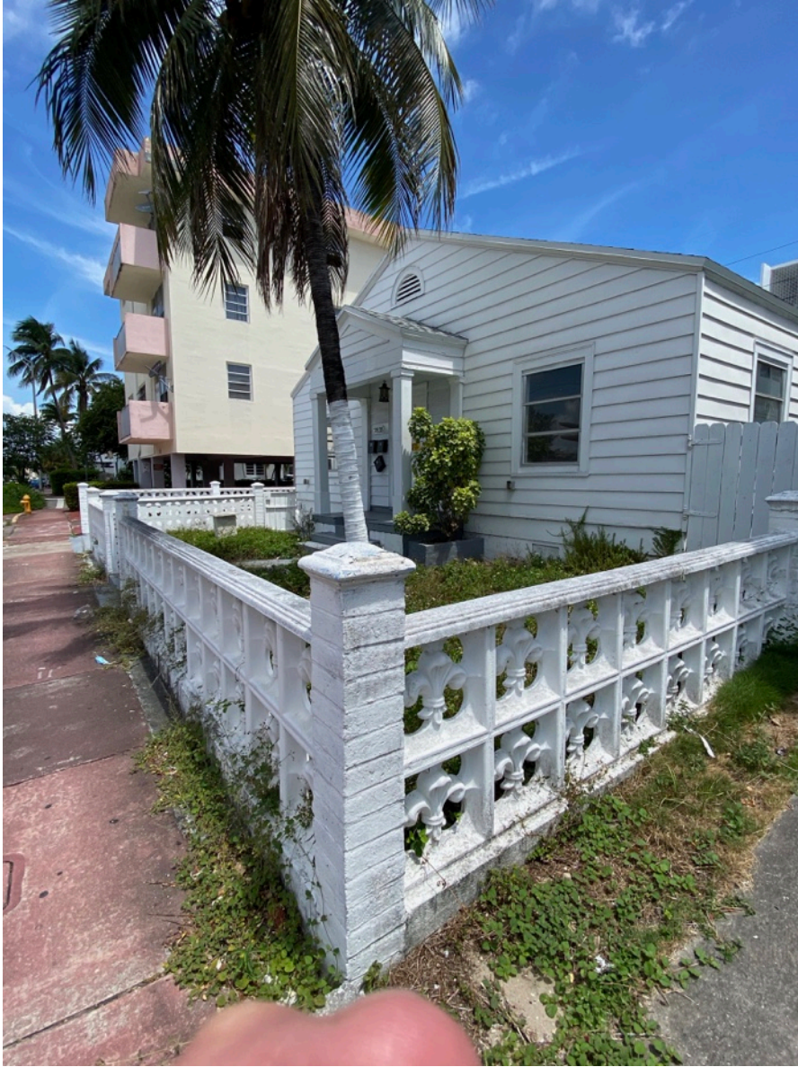
TOP PHOTO: FRONT YARD (11)
