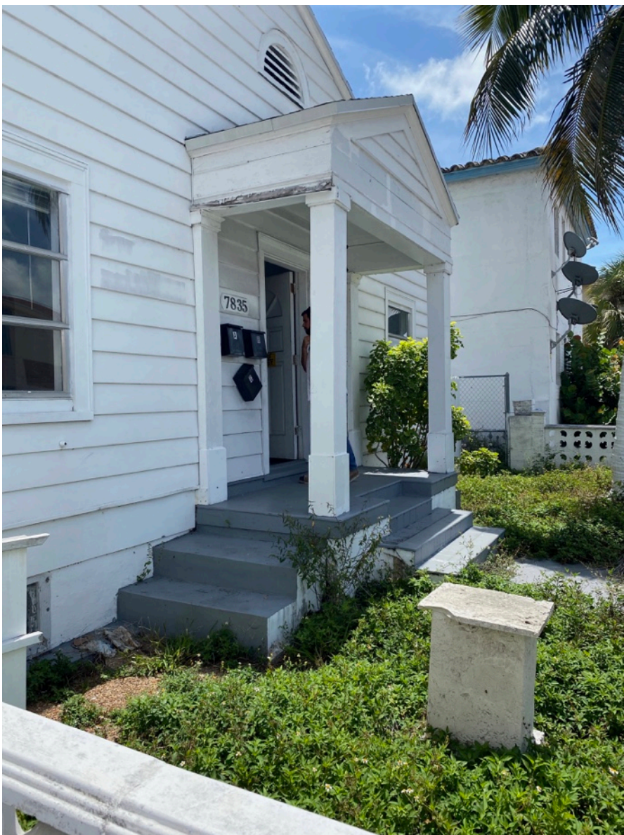
LOWER PHOTO: FRONT ENTRANCE (11)
