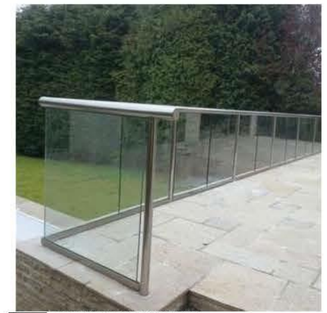
12 9/16" LAMINATED IMPACT GLASS GUARD RAIL SYSTEM (IMAGE FOR VISUAL REFERENCE ONLY)
