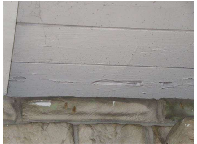
TERMITE DAMAGE
