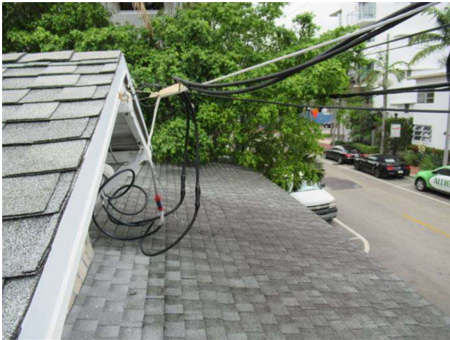
MAIN FEEDERS HEIGHT TO LOW
