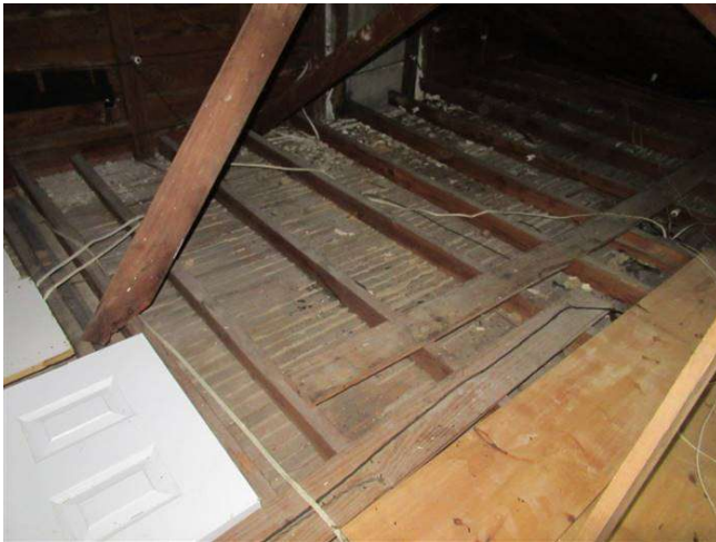
MISSING INSULATION
