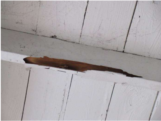
TERMITE DAMAGE
