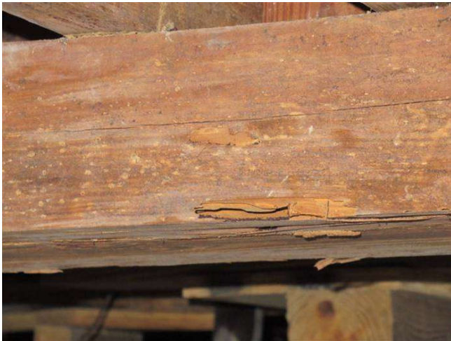
TERMITE DAMAGE/DROPPINGS
