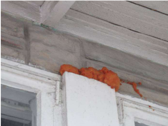
IMPROPERLY SEALED
