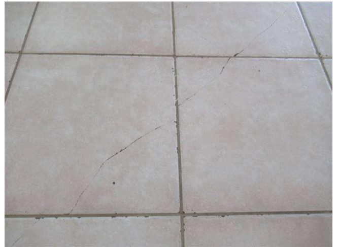
CHIPPED/CRACKED TILES
