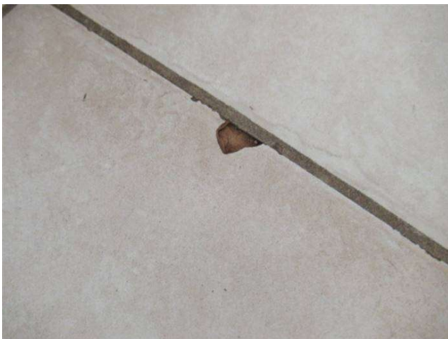
CHIPPED/CRACKED TILES
