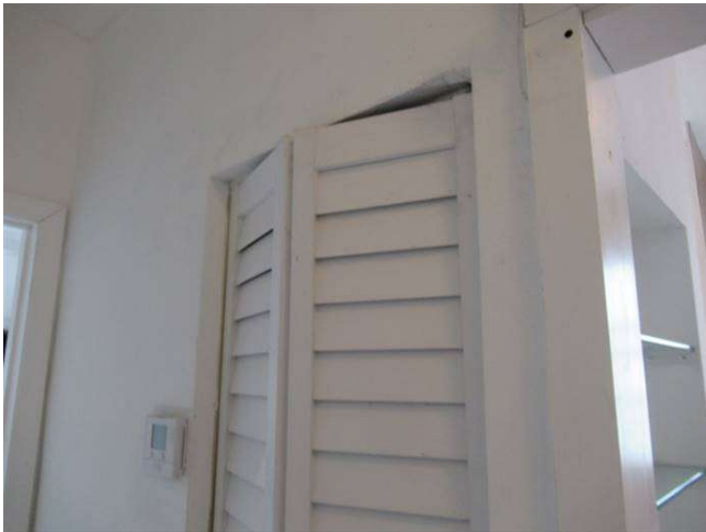
DAMAGED/LOOSE DOORS
