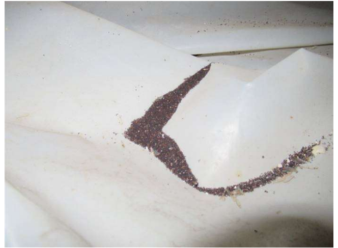
TERMITE DAMAGE/DROPPINGS
