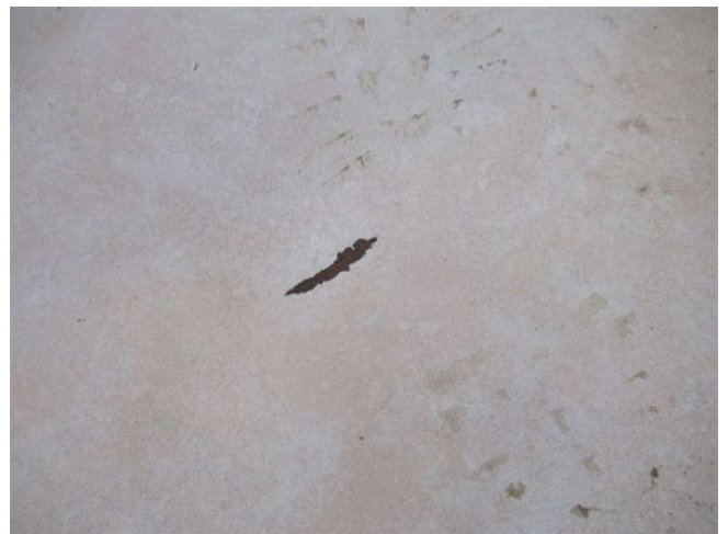
CHIPPED/CRACKED TILES
