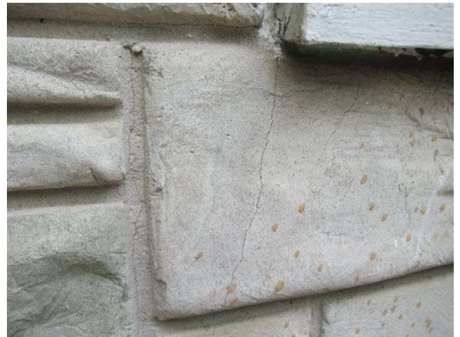
HAIRLINE CRACKS
