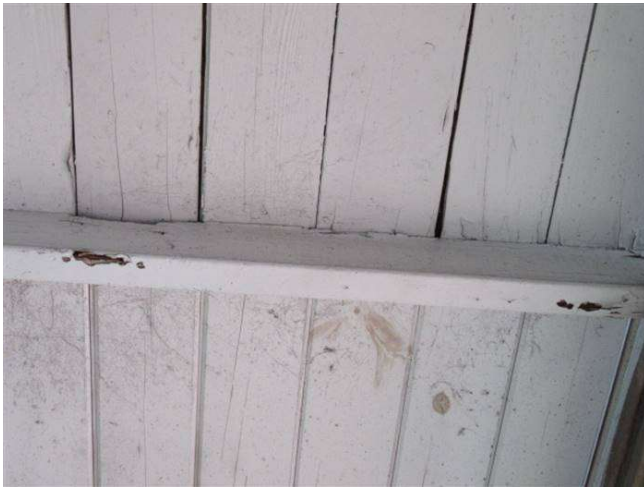
TERMITE DAMAGE
