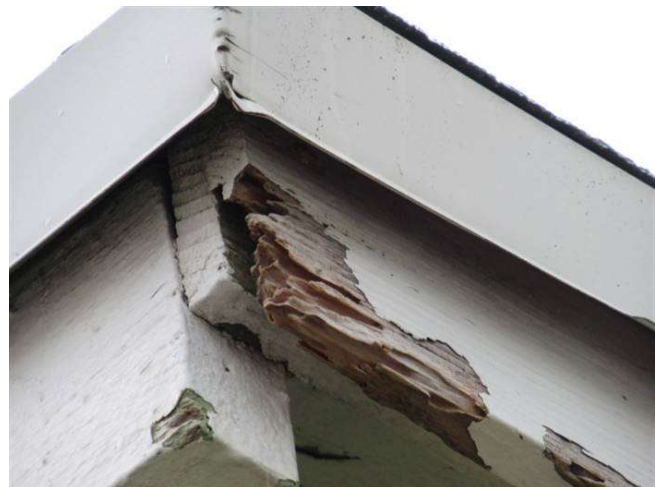
TERMITE DAMAGE
