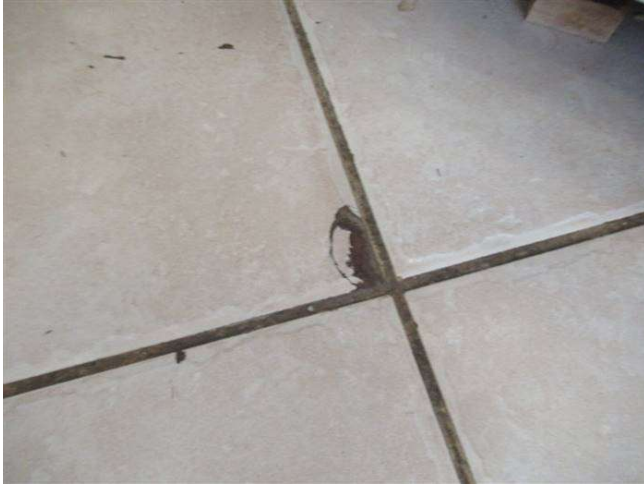
CHIPPED/CRACKED TILES
