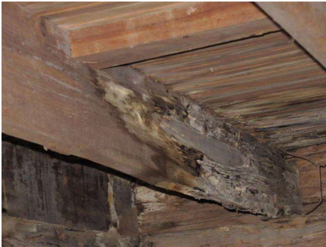
MOISTURE DAMAGE
