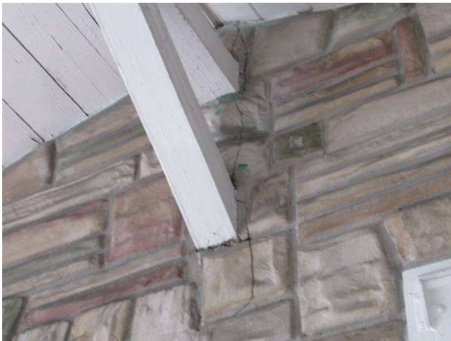
HAIRLINE CRACKS
