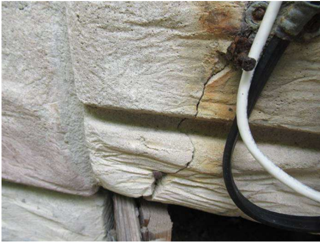
HAIRLINE CRACKS
