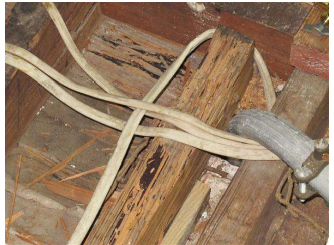
TERMITE DAMAGE
