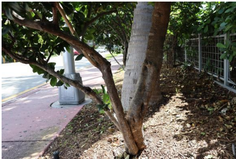
Note shaping and poor structure.
