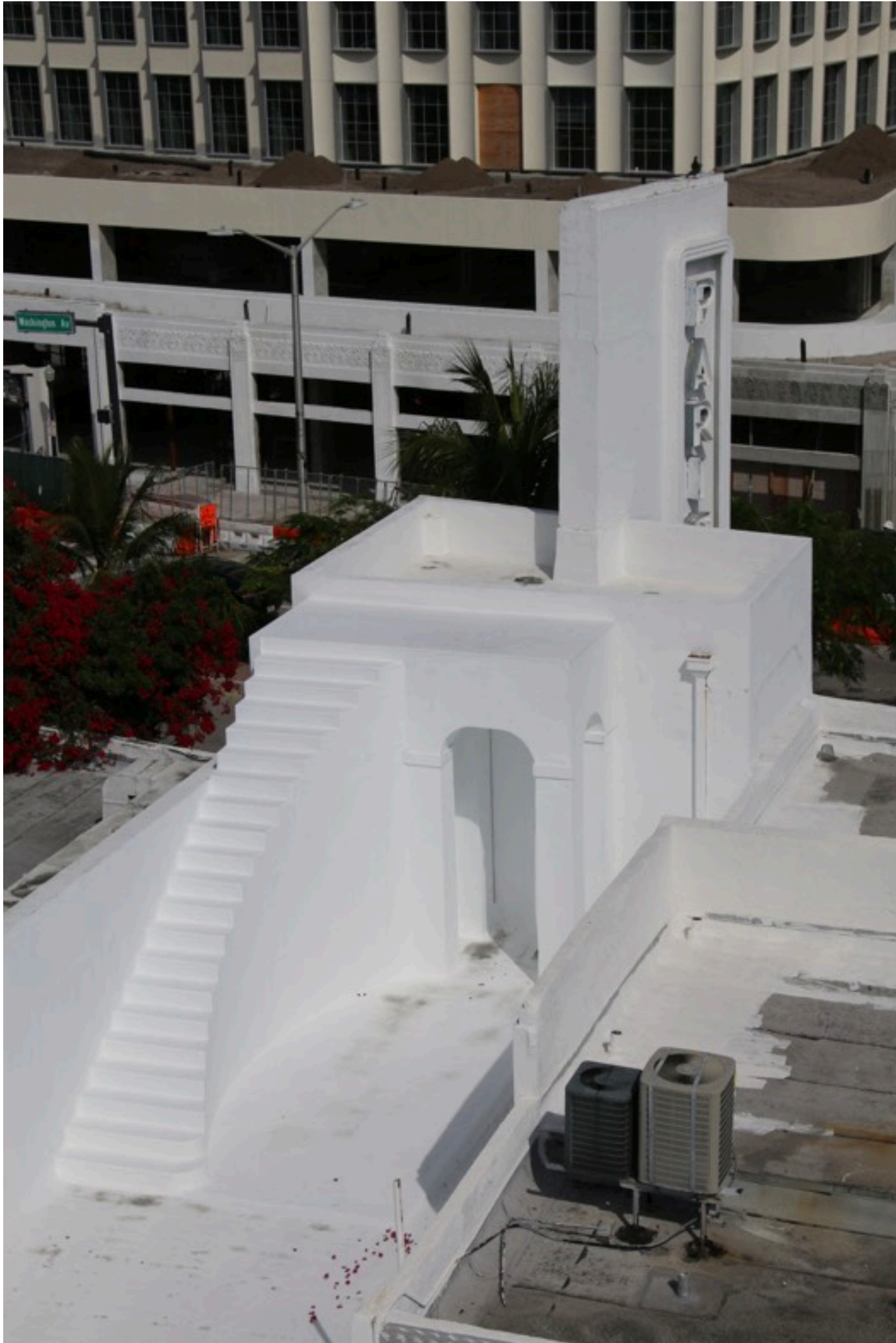
THE THEATER ROOFTOP CONTAINS MANY STRUCTURES AND STAIRS ESPECIALLY SUITABLE FOR PHOTOSHOOTS.. (23)
