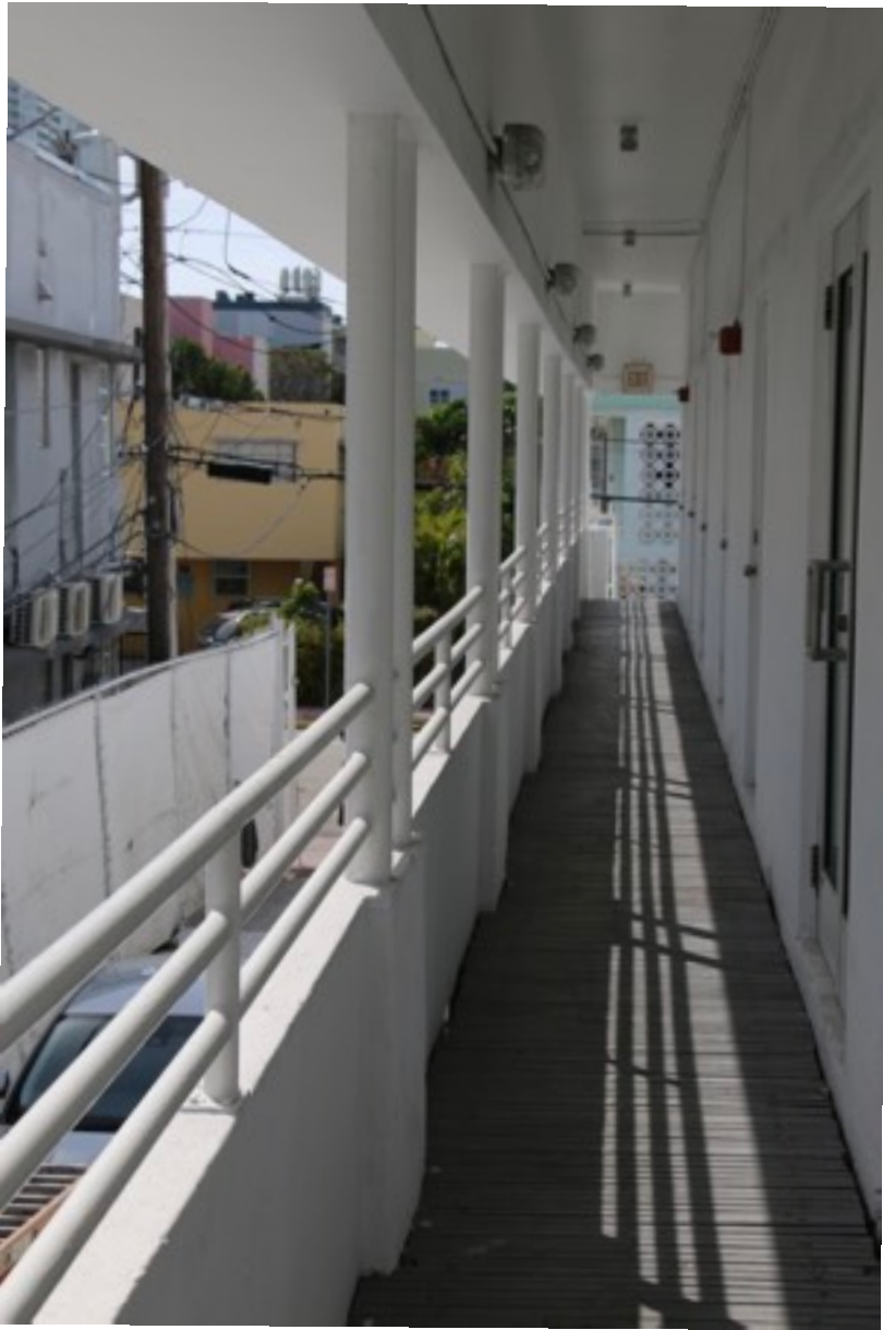
ABOVE: VIEW LOOKING WEST AT SECOND LEVEL PORTICO SPACE. (23)
