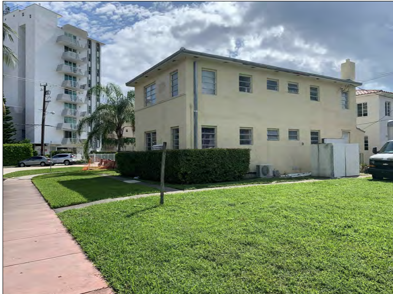
01 VIEW OF EAST NEIGHBOR PROPERTY A-06 SCALE:NTS
