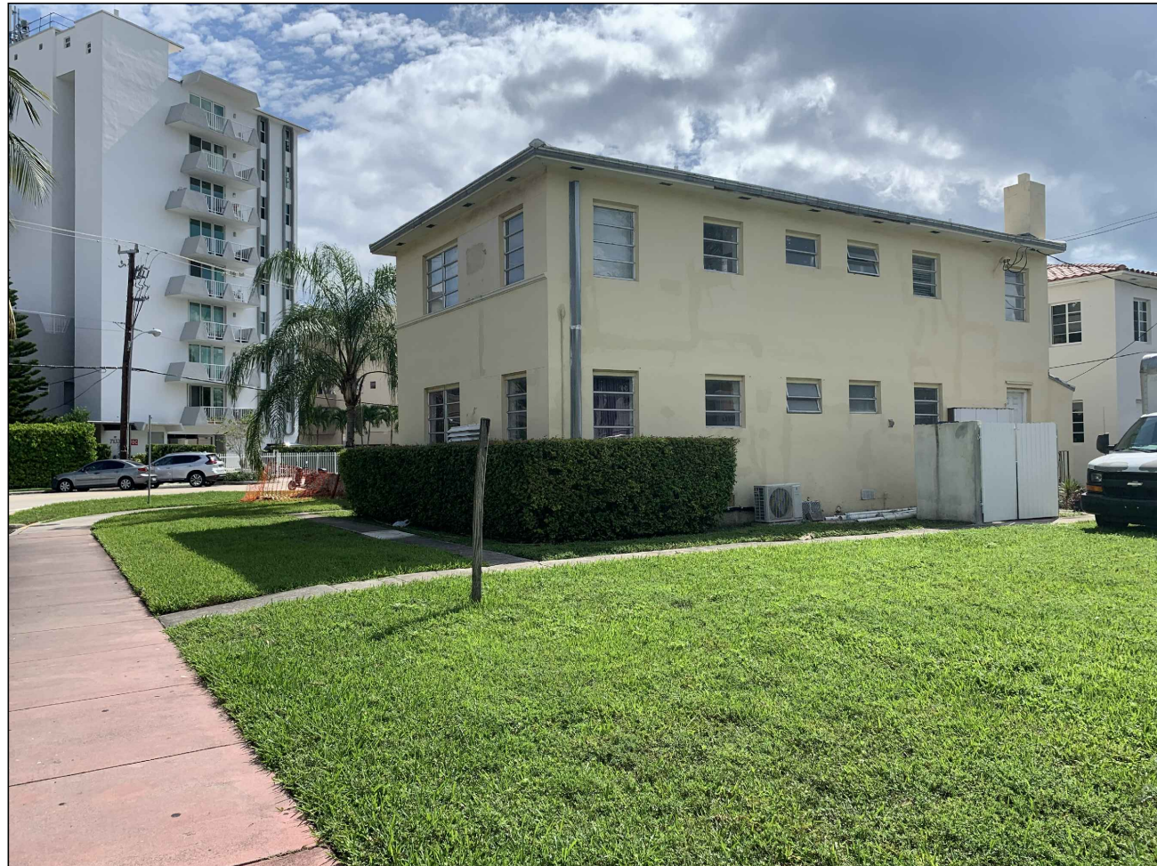
01 VIEW OF EAST NEIGHBOR PROPERTY A-06 SCALE:NTS
