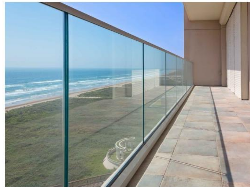
3 BALCONY RAILINGS - CLEAR GLASS A-31 SCALE:NTS
