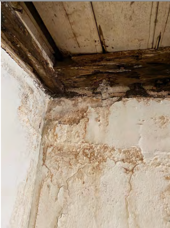
Photo 11 – Ceiling of covered patio
