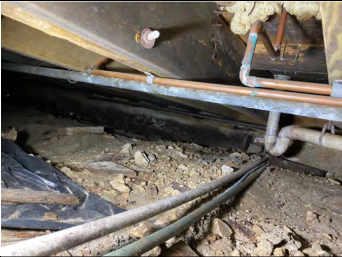
Photo 13 - Crawl space under house
