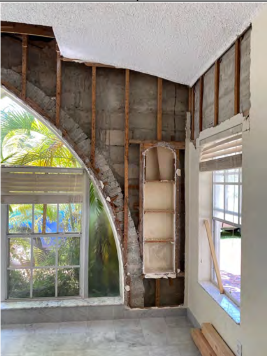
Photo 19 – Interior of west elevation
