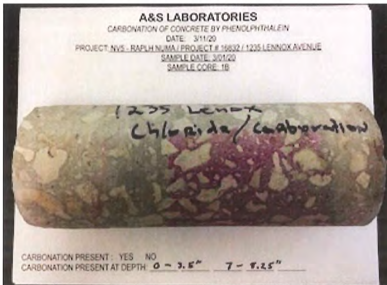
Figure 12: Carbonation Core Sample No. 1B: South Beam
