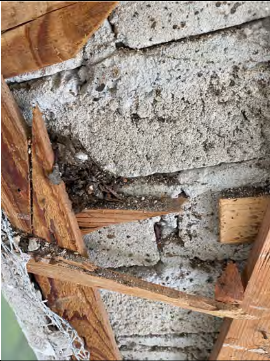
Photo 21 – Termite Damage and SMU
