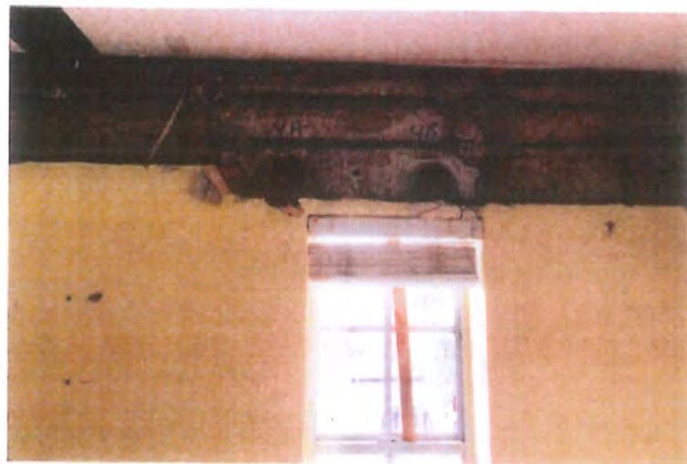
Figure 5: Core Location 4A, 4B: NW Beam
