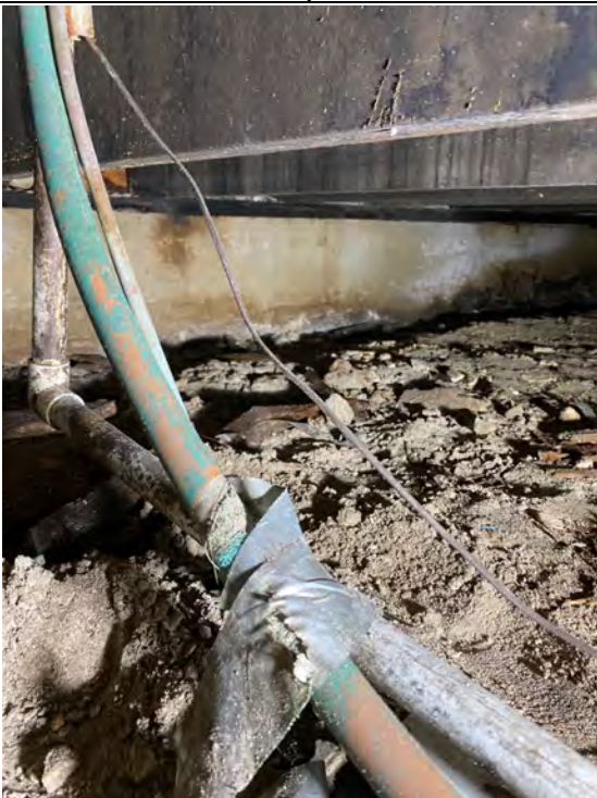
Photo 15 - Crawl space under house
