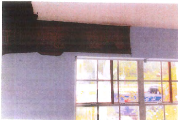
Figure 3: Core Location 2A, 2B: Ground Floor SW Beam
