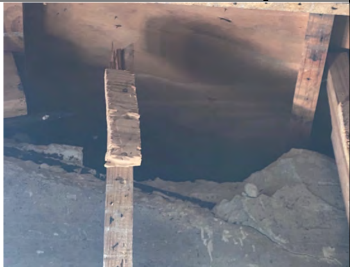
Photo 18 – Roof leaks damage
