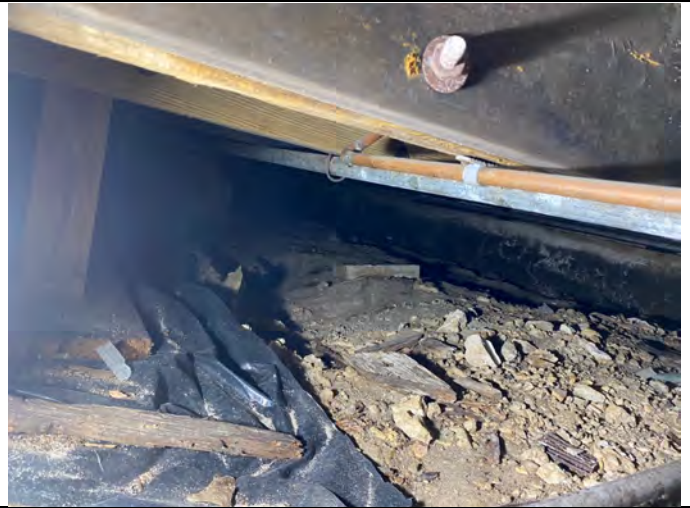
Photo 14 - Crawl space under house
