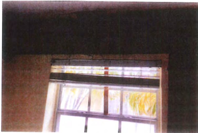
Figure 4: Core Location 3A, 3B: North Beam
