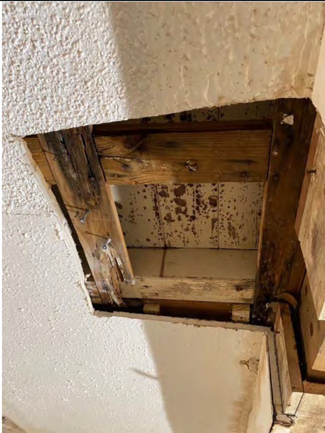
Photo 9 – Ceiling of covered patio
