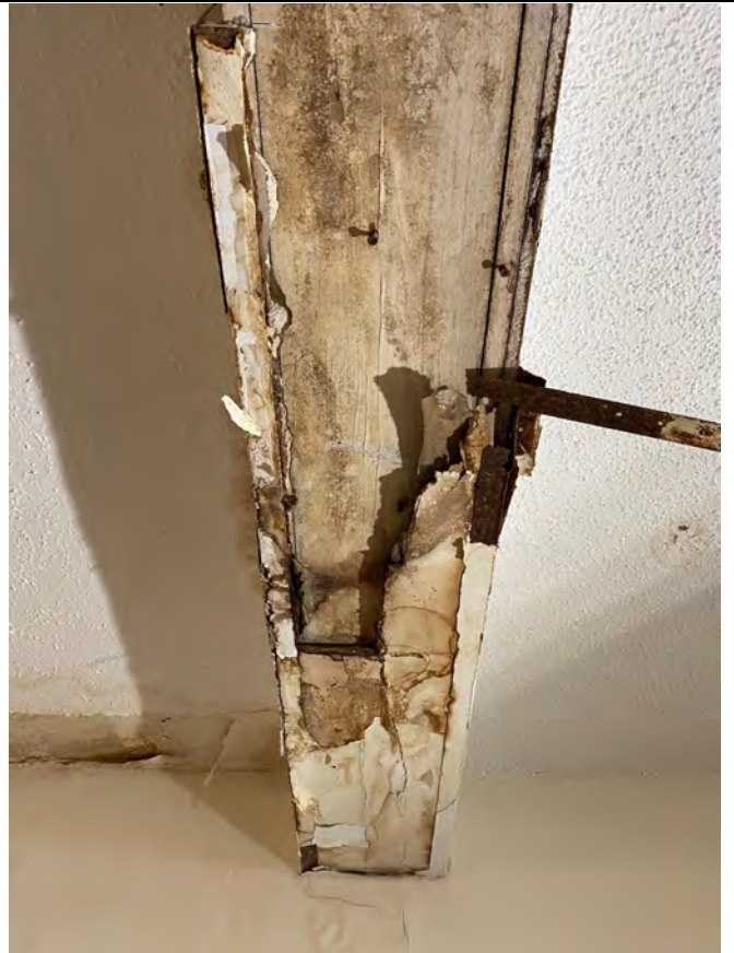
Photo 10 – Edge beam between covered patio and East addition
