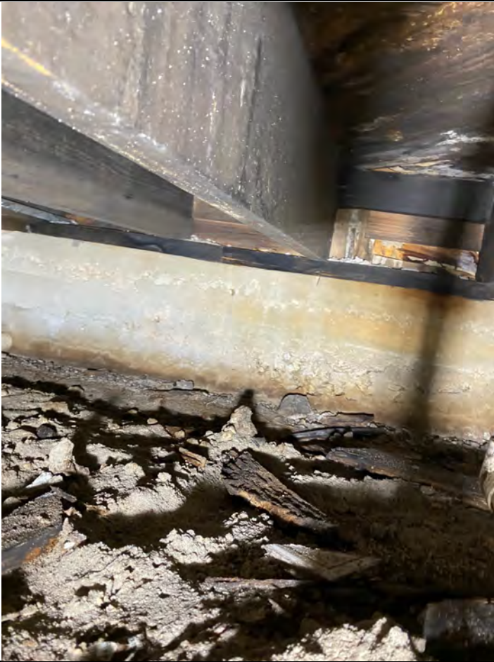
Photo 17 - Crawl space under house
