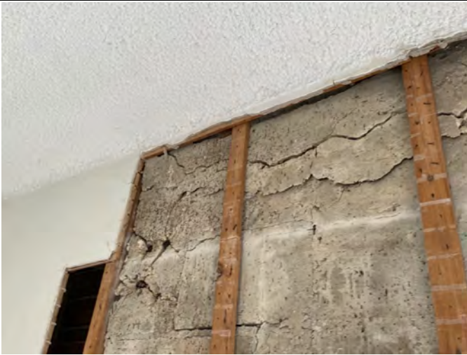
Photo 21 – Termite Damage and SMU
