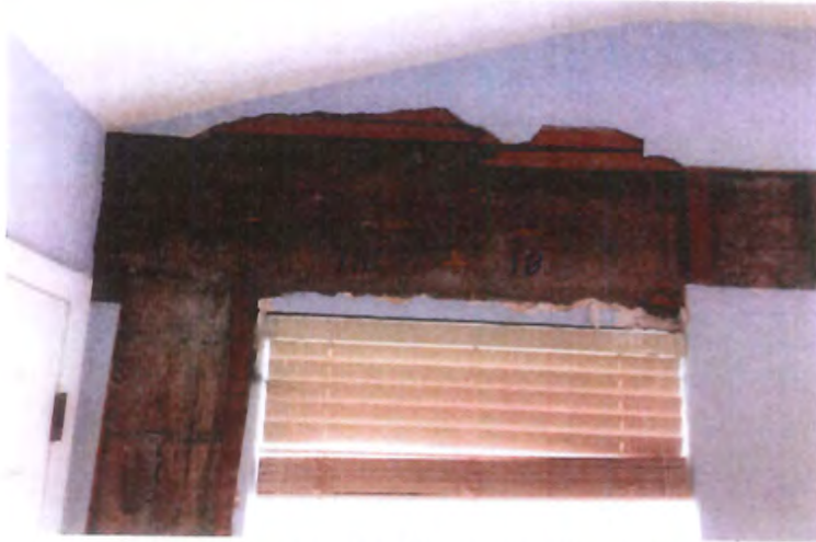
Figure 2: Core Location 1A, 1B: Ground Floor South Beam
