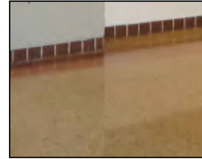
3 HISTORIC TERRAZZO FLOORING AND BASEBOARD
