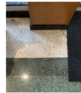
G BASEBOARD OVER NON-HISTORIC WOOD PANELING
