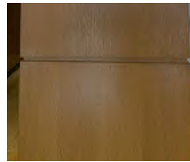
C EXISTING NON-HISTORIC WOOD PANELING
