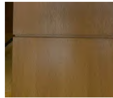
D EXISTING NON-HISTORIC WOOD PANELING
