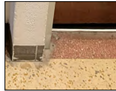
4 HISTORIC TERRAZO FLOORING AND BASEBOARD
