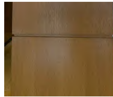
C EXISTING NON-HISTORIC WOOD PANELING
