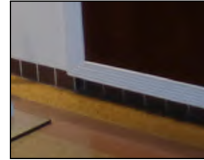
4 HISTORIC TERRAZO FLOORING AND BASEBOARD
