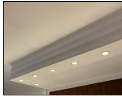
3 HISTORIC RECEPTION DROP-CEILING FEATURE
