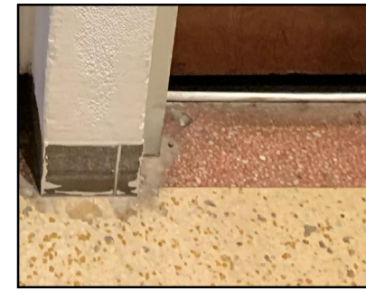
4 HISTORIC TERRAZO FLOORING AND BASEBOARD
