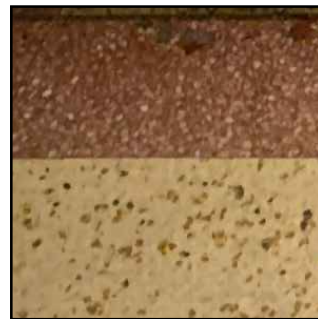
5 HISTORIC TERRAZO FLOORING
