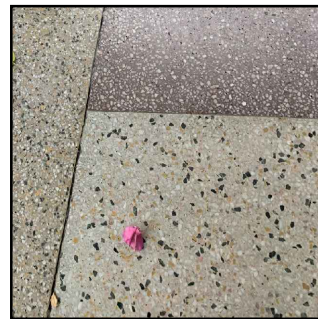
4 HISTORIC TERRAZO FLOORING
