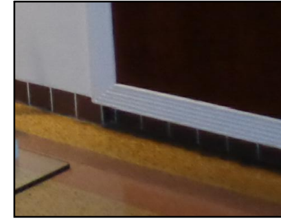
4 HISTORIC TERRAZO FLOORING AND BASEBOARD
