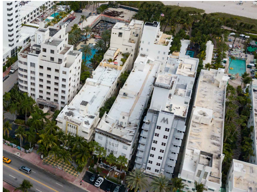
2 AERIAL VIEW TOWARD RALEIGH, RICHMOND & SOUTH SEAS ROOF
