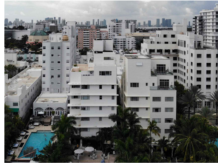
8 CLOSE UP VIEW TOWARD EAST FACADE OF RICHMOND & SOUTH SEAS
