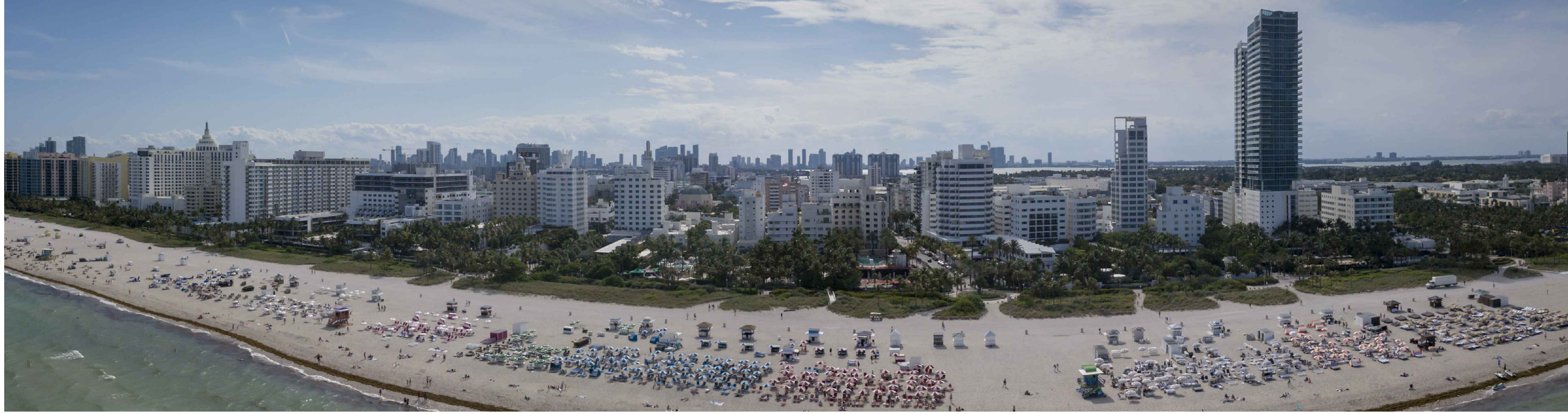
5 AERIAL VIEW FROM OCEAN TOWARD WEST
