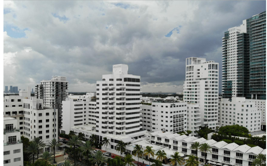
4 VIEW EAST TOWARD NORTHWEST
