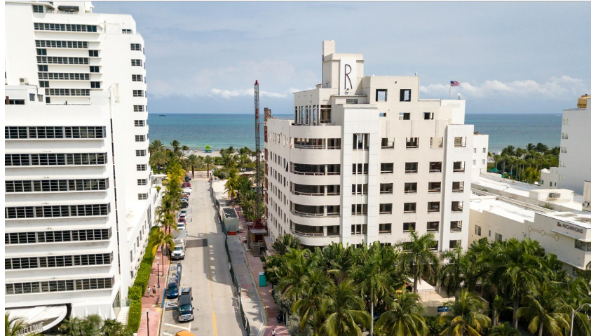
4 AERIAL VIEW TOWARD EAST - 18TH STREET
