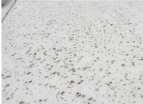
Concrete with Salt Finish
