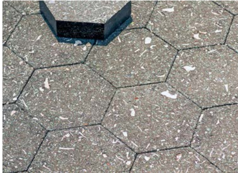
Asphalt paver with shell aggregate
