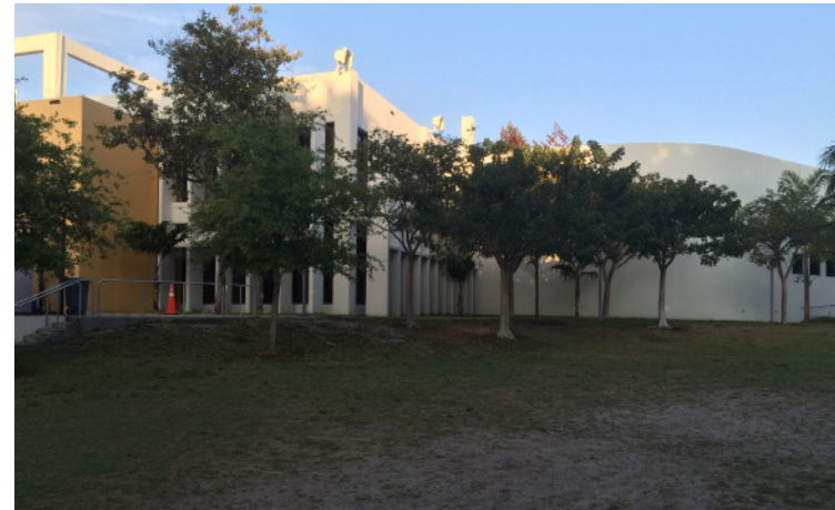
6. Northeast corner of site facing North. ( Youth Center )
