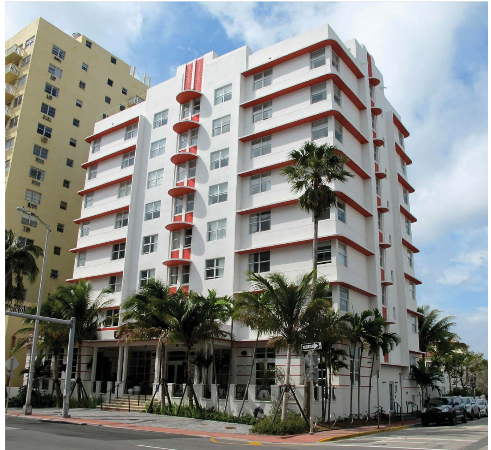
2 BUILDING C: POST-RESTORATION CONDITION (2019) SCALE: N.T.S.
